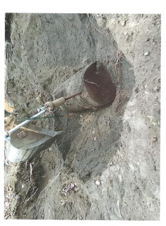
Tank was located under 44" of native soil. Underground Storage Tank was 45.5" x 6'L (500-Gallons). There was no visible holes in tank.
