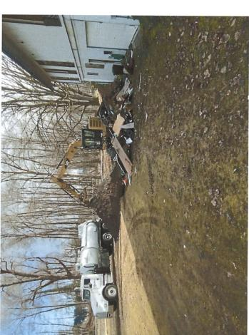
Northern Environmental LLC employee triple rinsed the tank for any residual oil. Tank must be properly cleaned to dispose of.
