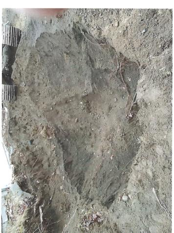
After the tank was removed by Sita Enterprises, a soil sample was taken in pit are at 8.5'. Then sent to Libby Environmental for lab analysis.
