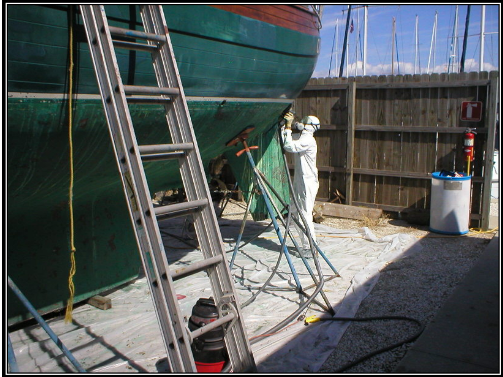
Figure 4.22. Drop Cloth Used During Hull Sanding.
