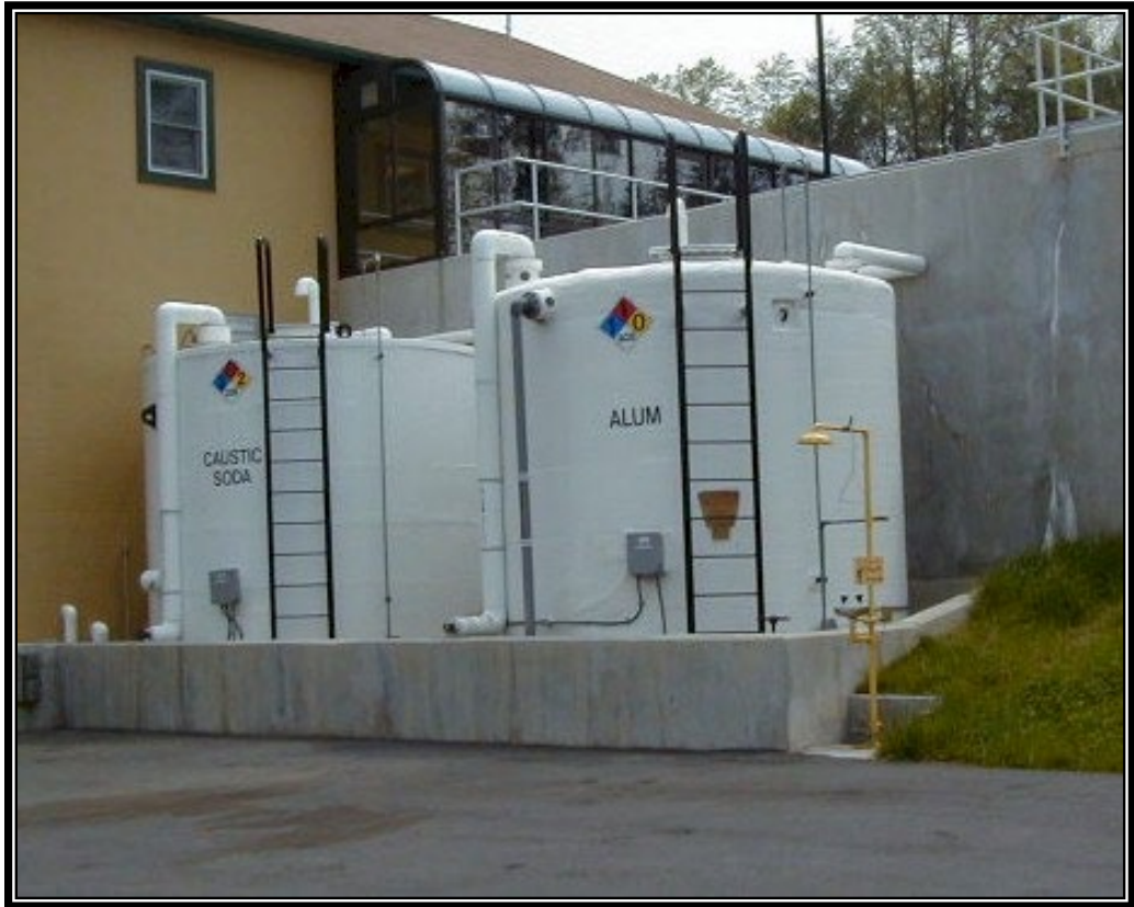
Figure 4.19. Aboveground Storage Tanks with Secondary Containment.
