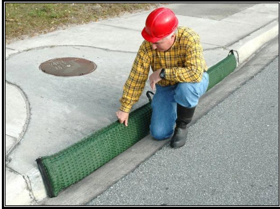
Figure 4.20. Commercially Available Gutter Guard Being Replaced.
