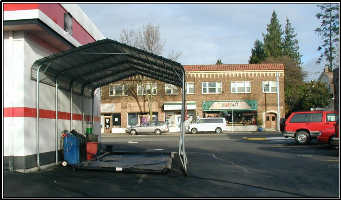
(Photo courtesy of Seattle Public Utilities)
