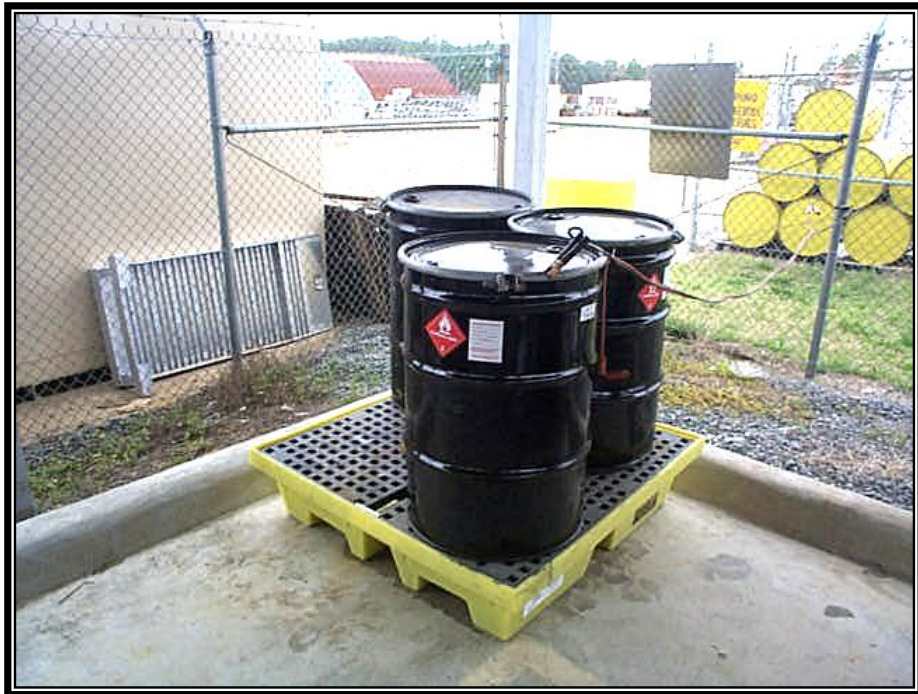
Figure 4.17. Temporary Secondary Containment.
