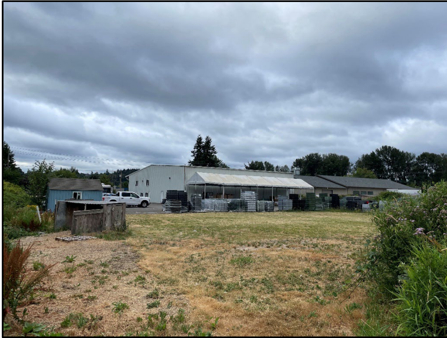
Figure 3. Overview of project area with CIMCO sales facility in background – view south/southwest.
