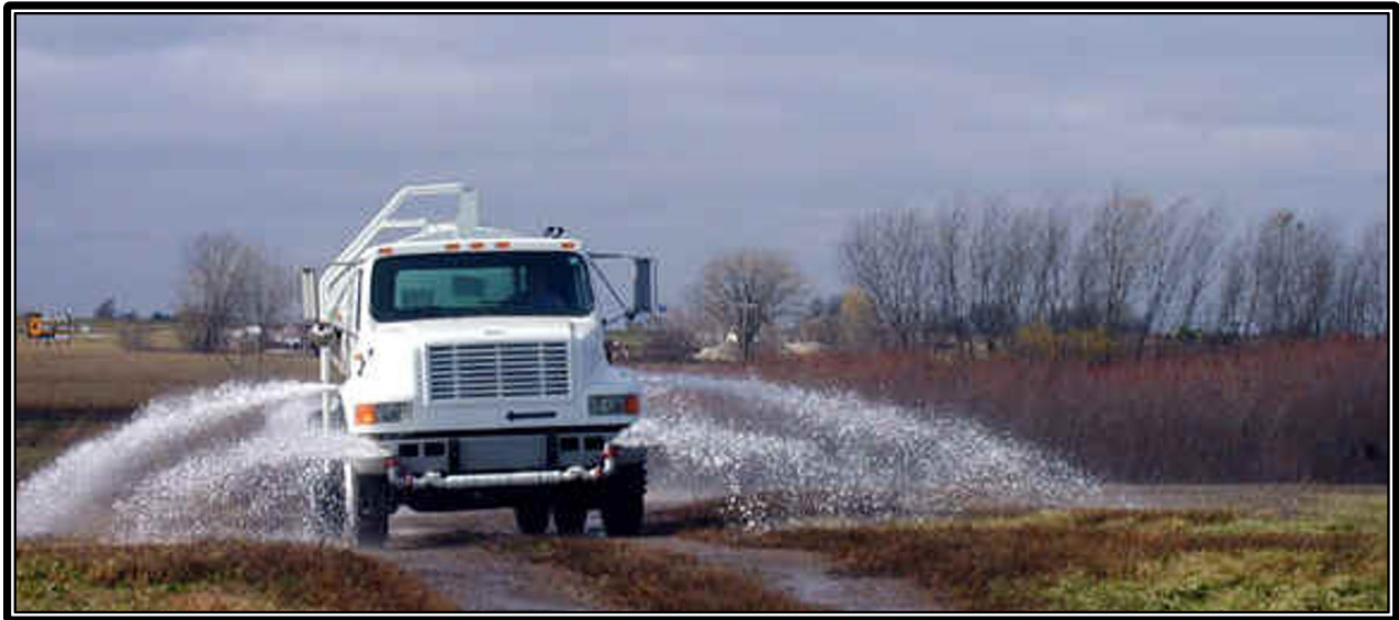
Figure 4.21. Dust Suppression by Water Spray.
