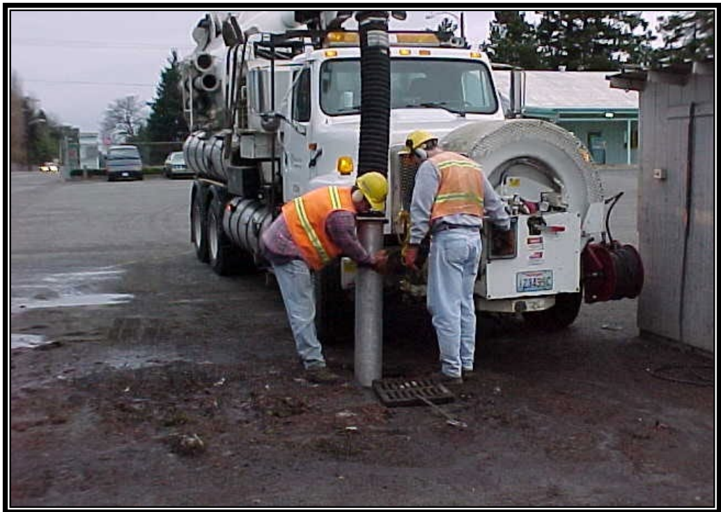
Figure 4.23. Catch Basin Cleaning with a Vacuum Truck.
