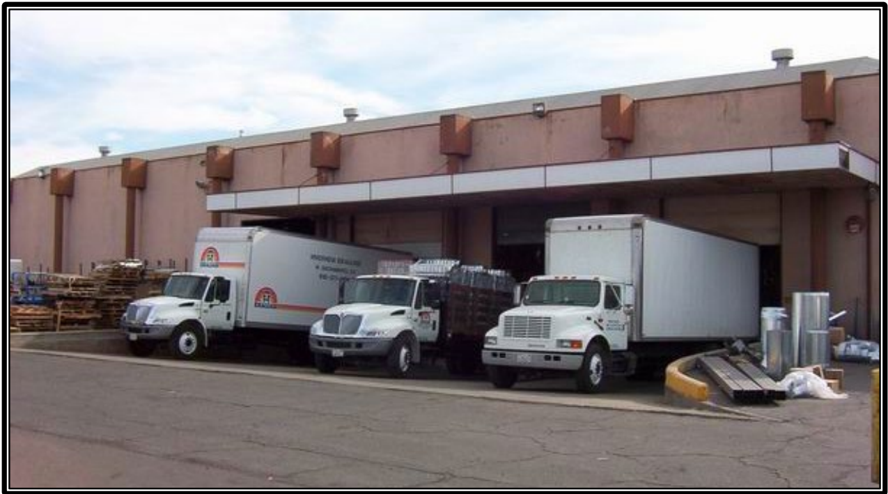
Figure 4.5. Loading Docks with an Overhang to Prevent Material Contact with Rainwater.
