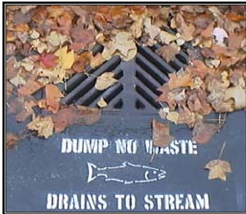
(Photo courtesy of Seattle Public Utilities)
