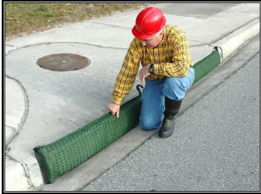
Figure 4.20. Commercially Available Gutter Guard Being Replaced.
