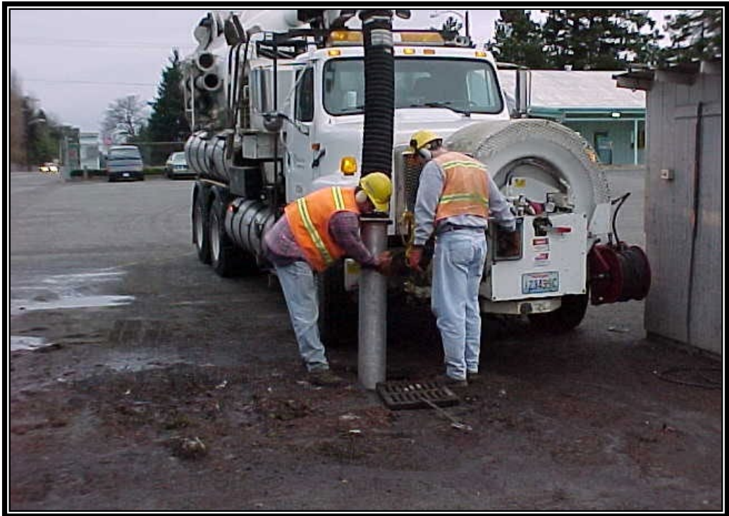
Figure 4.23. Catch Basin Cleaning with a Vacuum Truck.
