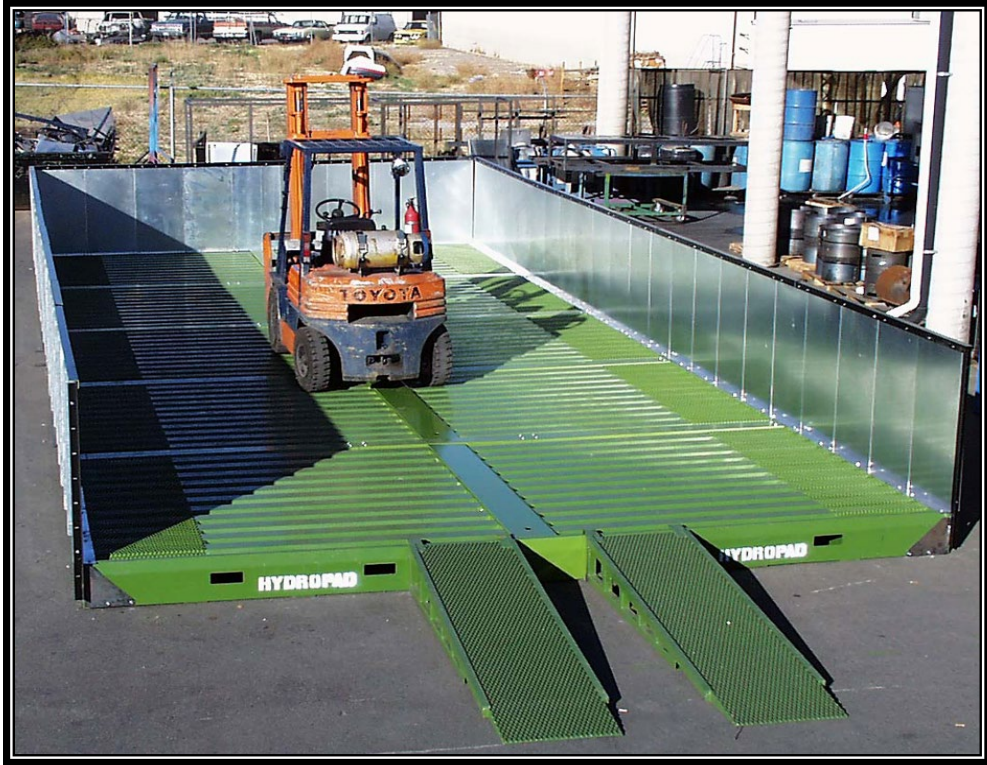
Figure 4.2. Uncovered Washing Area for Tools, Engines, Equipment, and Portable Objects, with Drains to a Sanitary Sewer, Process Treatment, or a Dead-End Sump.
