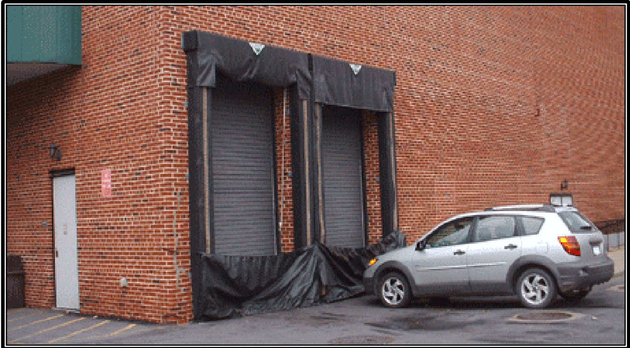
Figure 4.6. Door Skirts to Enclose the Trailer End of a Truck to Prevent Material Contact with Rainwater.
