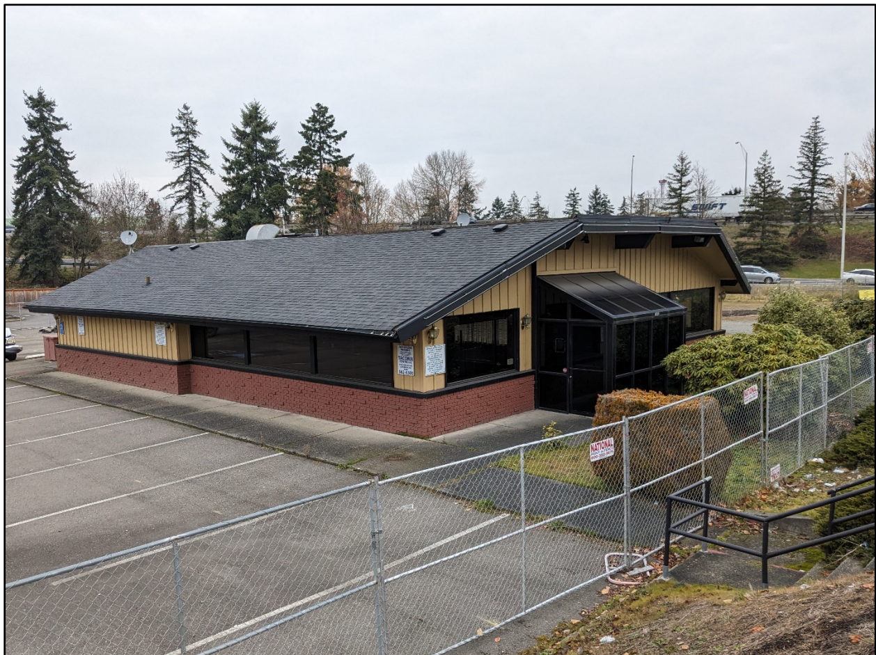
Figure 9. Project overview showing recently closed Jason's Restaurant, view NW.
