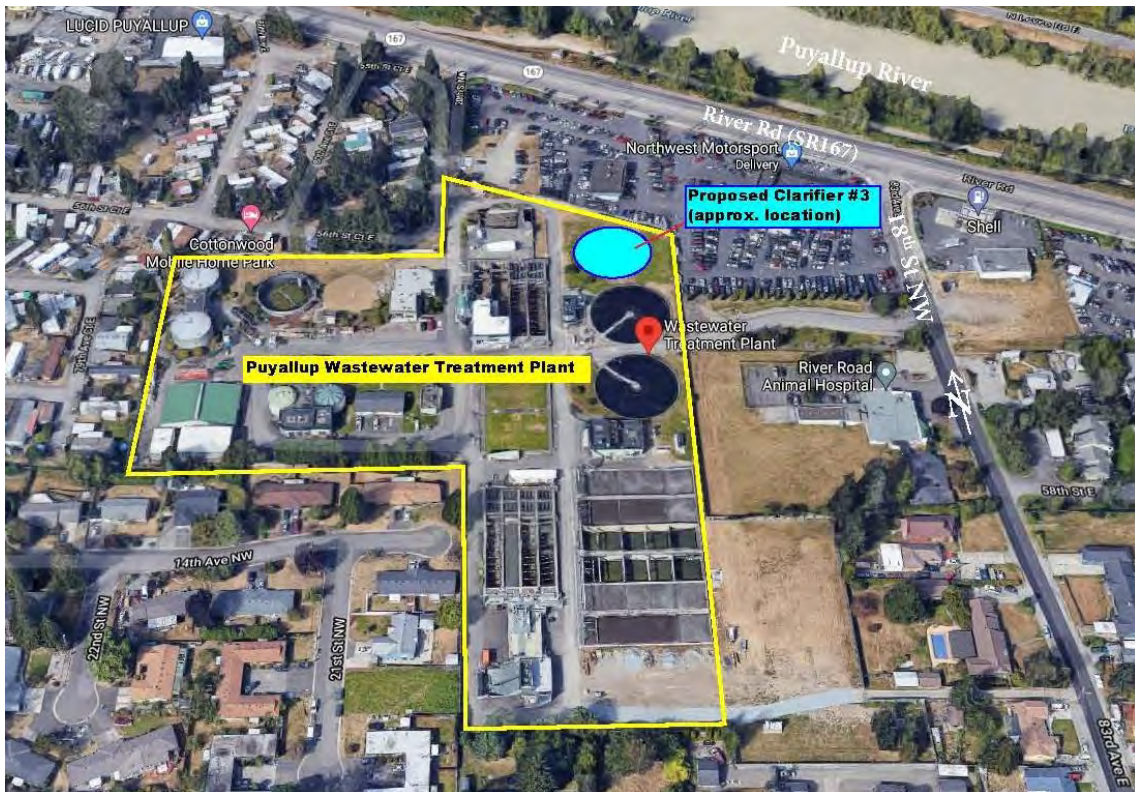
Plate 1. Existing Puyallup Wastewater Treatment Plant (modified based on Google map)
