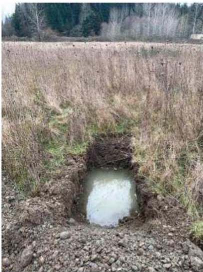
Water in Test Pit on March 5, 2021. Test pit was excavated in NE portion of site on March 4, 2021.
