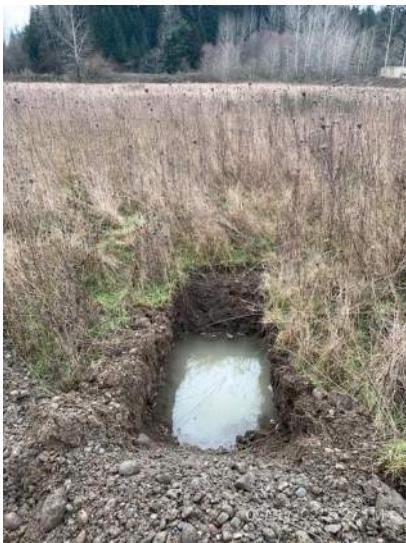
Water in Test Pit on March 5, 2021. Test pit was excavated in NE portion of site on March 4, 2021.
