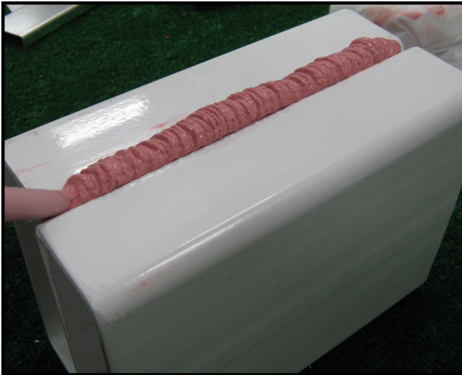
Caulk split with Joint & Seam caulking.
