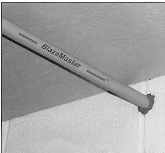
2 Hour Fire Rated Through Penetration Firestop for Single Plastic Pipe through Concrete Floors or Walls using BlazeMaster® Caulk & Walk®
