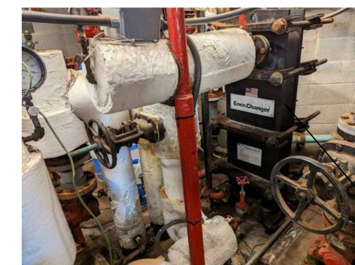
3 Heat Exchanger 2 Location SCALE: NONE
