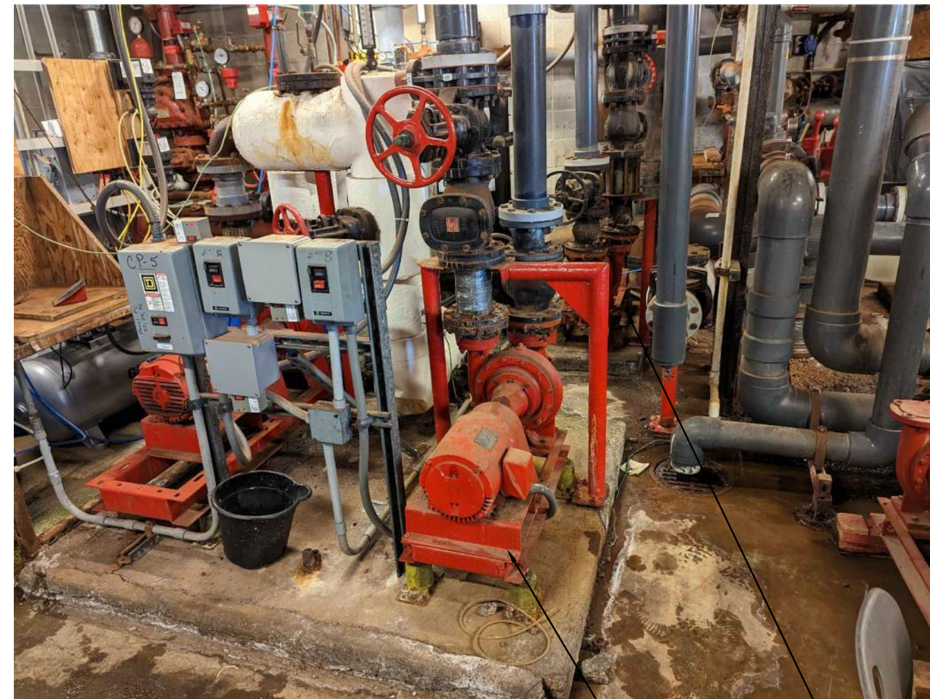
1 Heat Exchanger Pump Location SCALE: NONE
