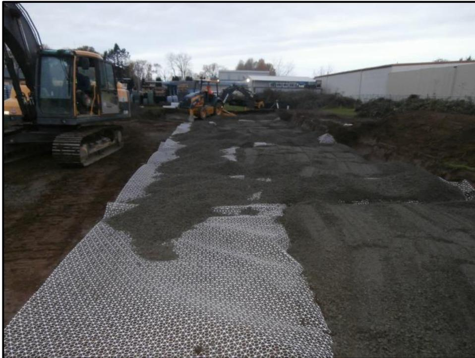
**Figure 12.** Photograph of gravel layer over structural fabric, facing west.
