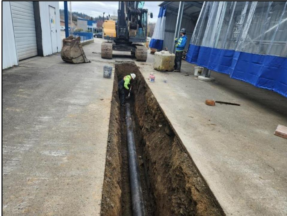
**Figure 54.** Photograph of the excavated trench with water pipe laid, view south
