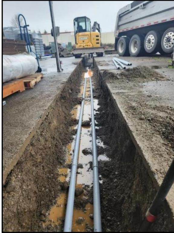
**Figure 21.** Overview of completed trench at site, facing north.
