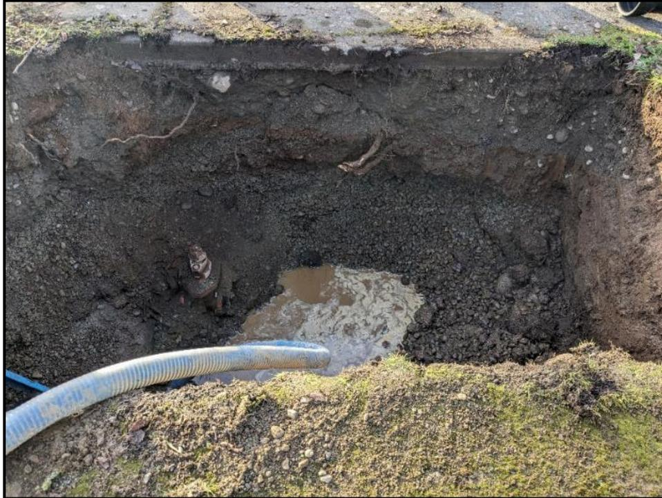
**Figure 35.** Photo of trench for fire hydrant replacement with high water table evident, plan view.
