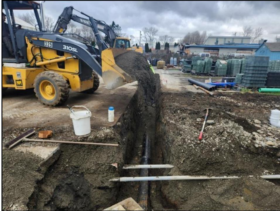
**Figure 52.** Photograph of gravel being used to fill in the excavated trench, view west
