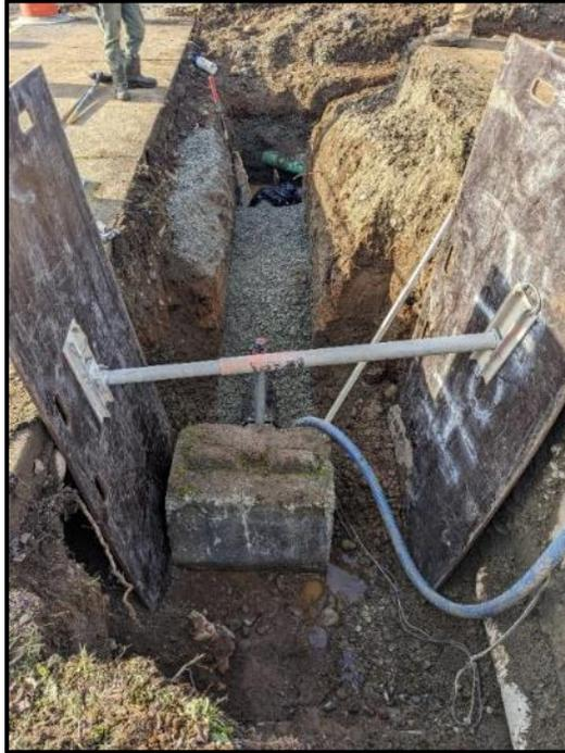
**Figure 36.** Photo of water line installation at fire hydrant with 90-degree bend in background, plan view, facing west.
