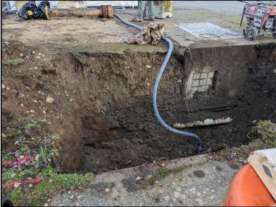
**Figure 27.** Photo of trench for fire hydrant replacement, view northeast.
