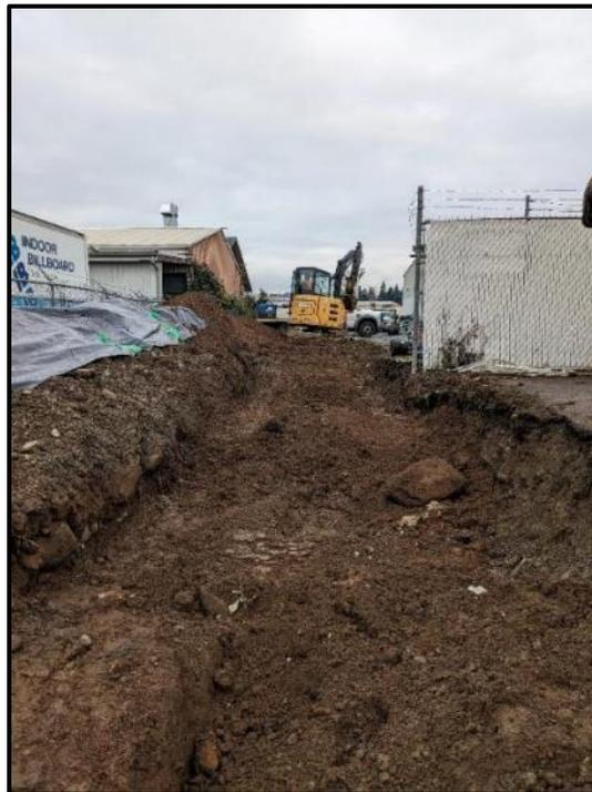
**Figure 41.** Photo of trench after backfilling, taken at 90-degree bend, view north.
