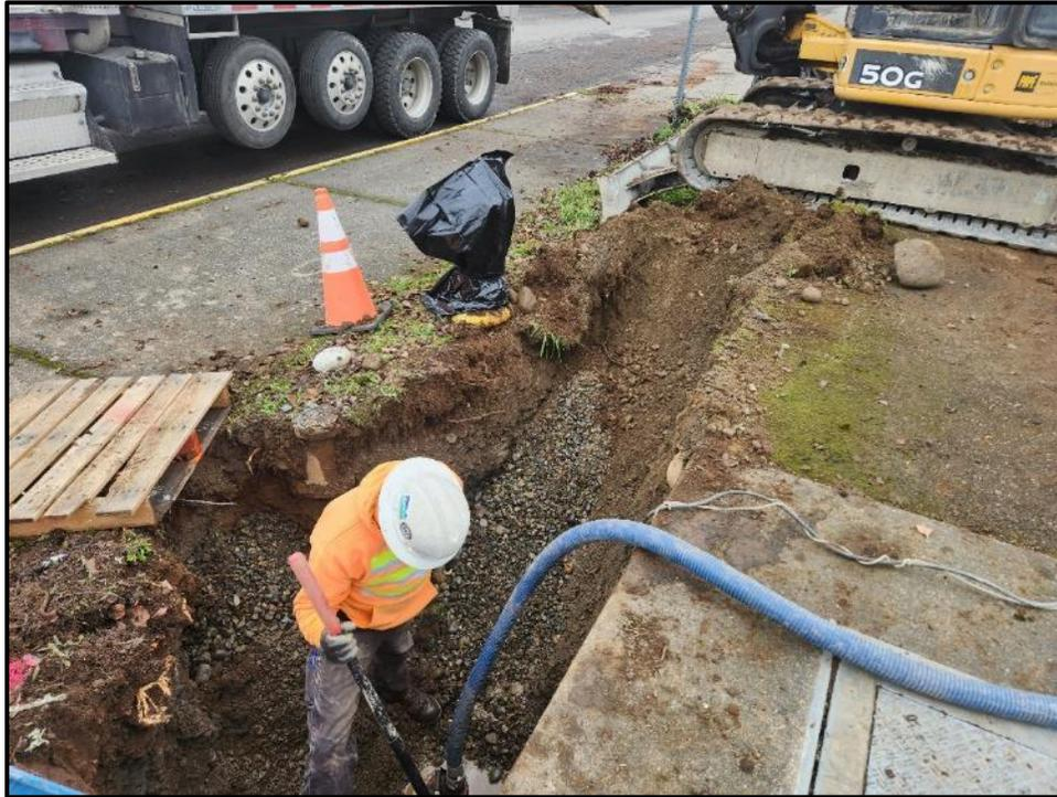
**Figure 24.** Photo of water table exposed, plan view facing southwest.
