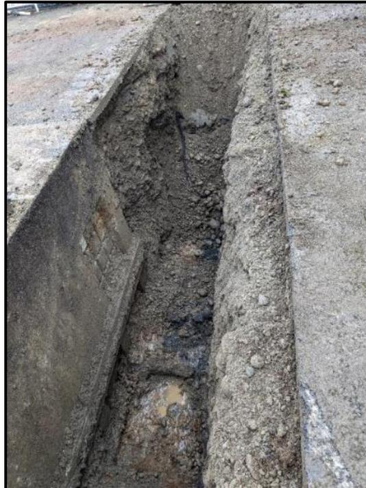
**Figure 45.** Photo of trench with asphalt aggregate backfill mixed in with disturbed soil, plan view.
