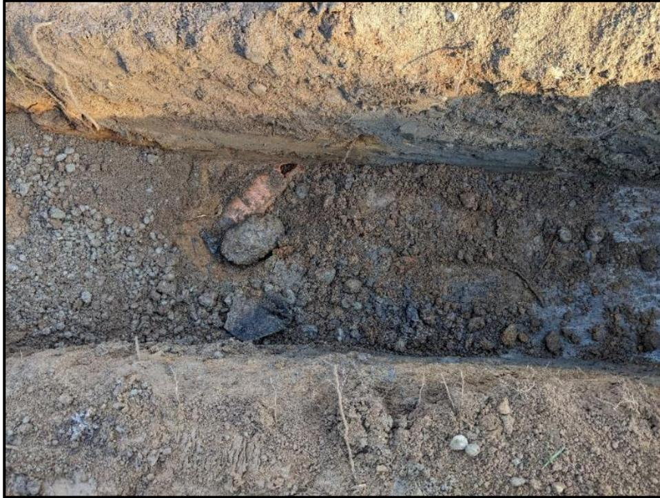
**Figure 32.** Photo of trench at exposed “dry” (abandoned) terracotta pipe, plan view.
