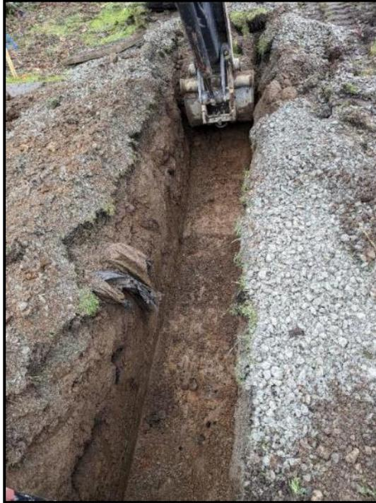
**Figure 38.** Photo of trench floor with excavator working in background, plan view, aspect north.
