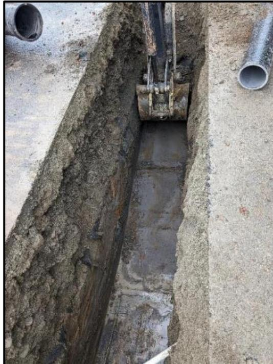
**Figure 46.** Photo of excavation activities with soil variations evident on trench floor, plan view.
