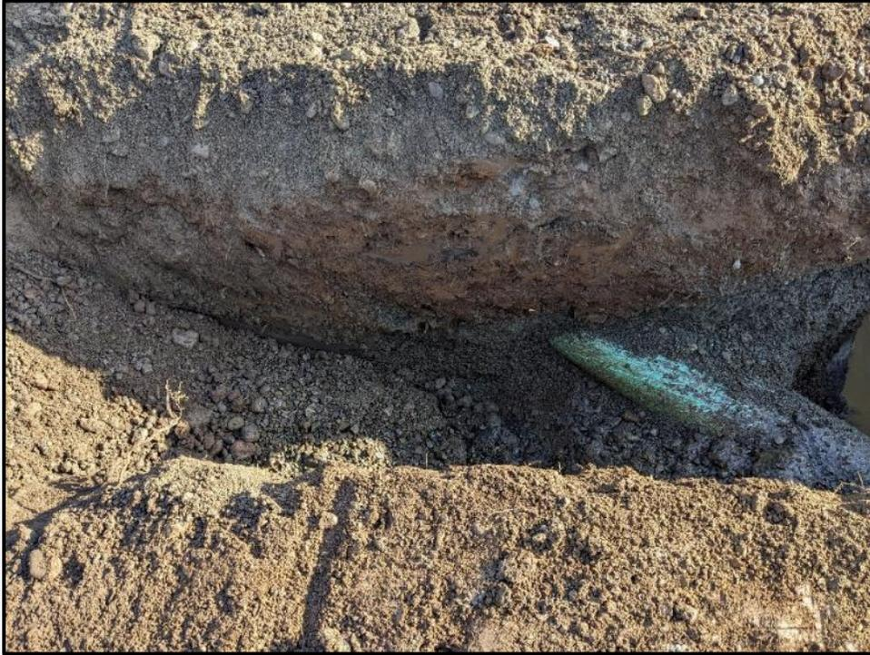
**Figure 34.** Photo of 90-degree bend with storm line exposed, plan view, facing east.
