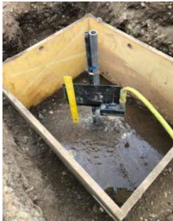
Test Pit Pre-soak at 12-inches
