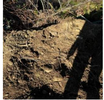
Backfill Test Hole
