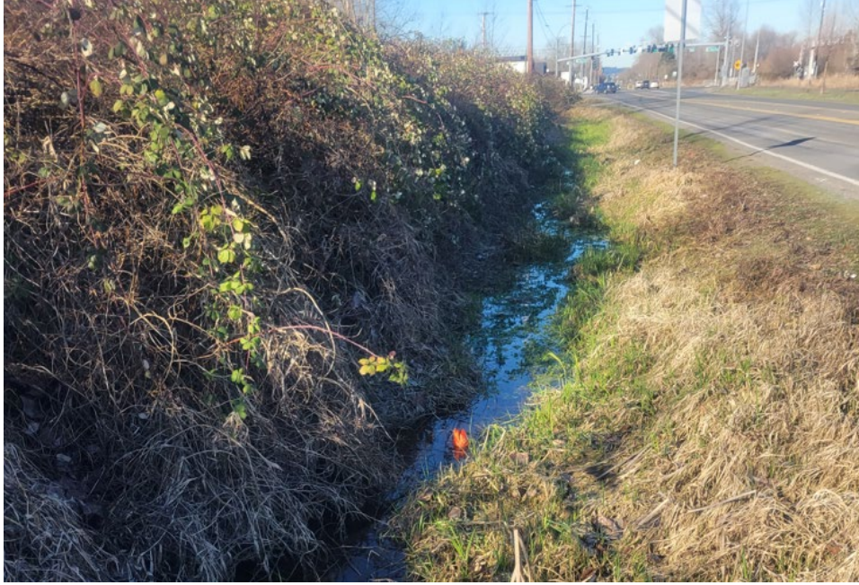
Typical degraded conditions of Stream Z within ROW of East Pioneer Avenue
