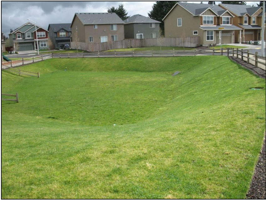
Example of a Manicured Detention Pond
