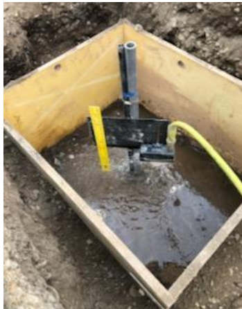
Test Pit Pre-soak at 12-inches
