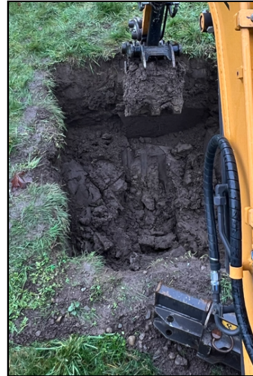
Overexcavate to Verify Groundwater Mounding
