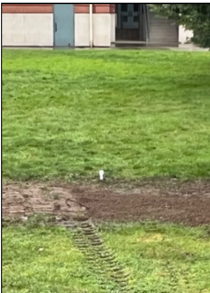
Backfill and Install Groundwater Monitoring
