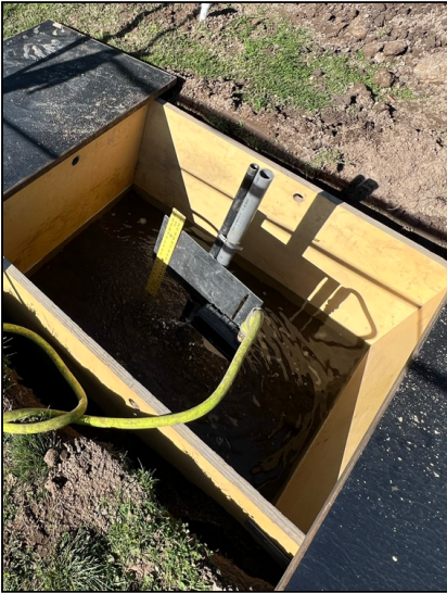
3-feet x 4-feet x 2-feet PIT and Pre-Soak
