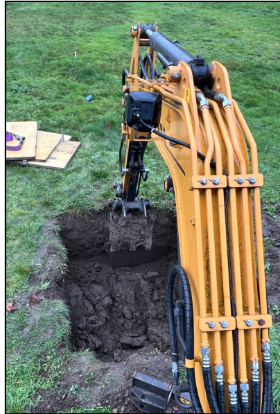
Overexcavate to Verify Groundwater Mounding
