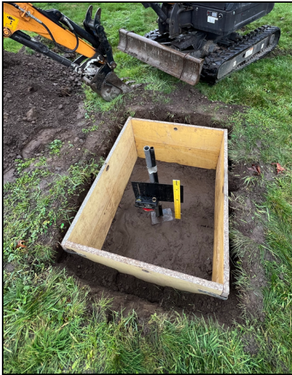
3-feet x 4-feet x 2-feet PIT
