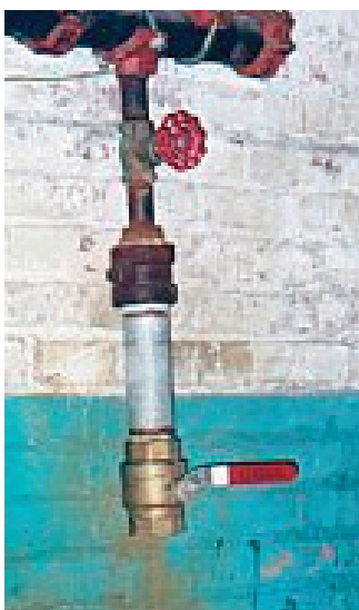
Example of a field generated drum drip with multiple fittings and pipe nipples. NOTE: the example shows seven make-ups.
