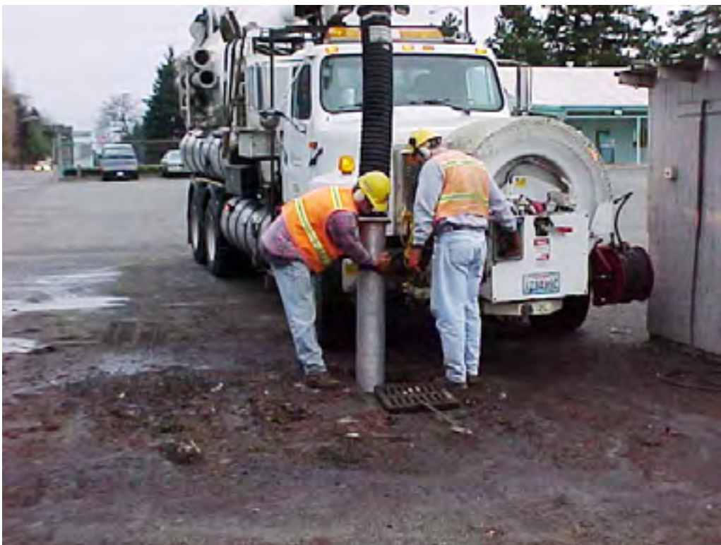
Figure 4.23. - Catch Basin Cleaning with a Vacuum Truck.
