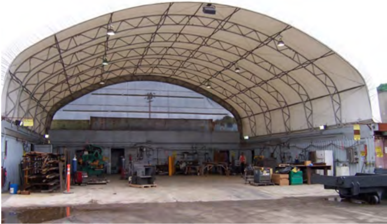
Figure 4.11. - Structure Used to Cover Manufacturing Operations.
