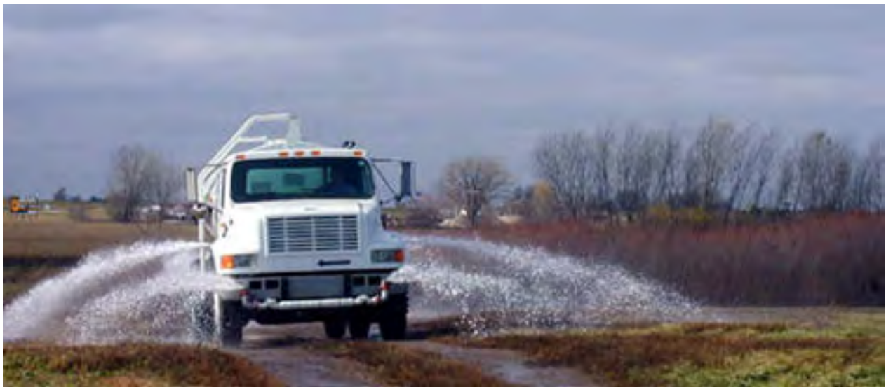
Figure 4.21. - Dust Suppression by Water Spray.
