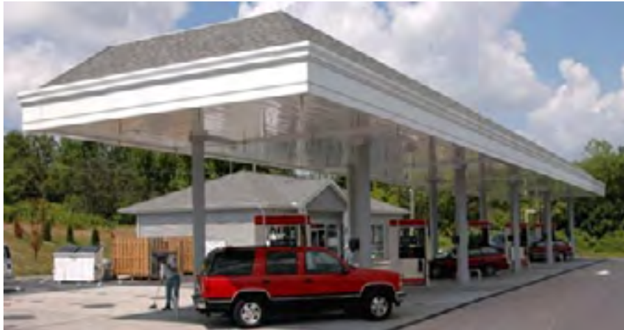
Figure 4.7. - Roof at Fueling Island to Prevent Stormwater Runon.
