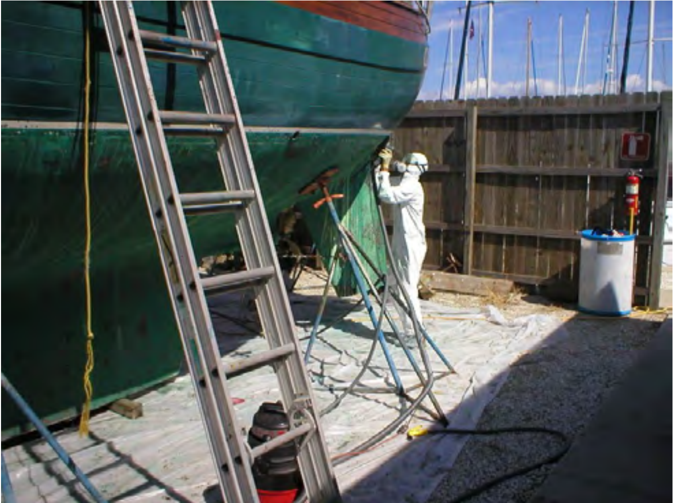
Figure 4.22. - Drop Cloth Used During Hull Sanding.
