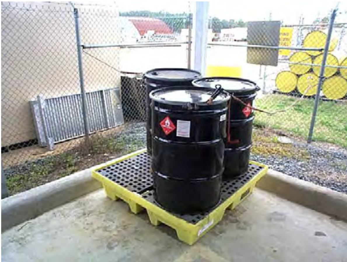
Figure 4.17. - Temporary Secondary Containment.
