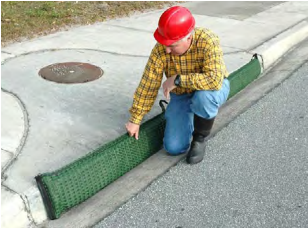
Figure 4.20. - Commercially Available Gutter Guard Being Replaced.
