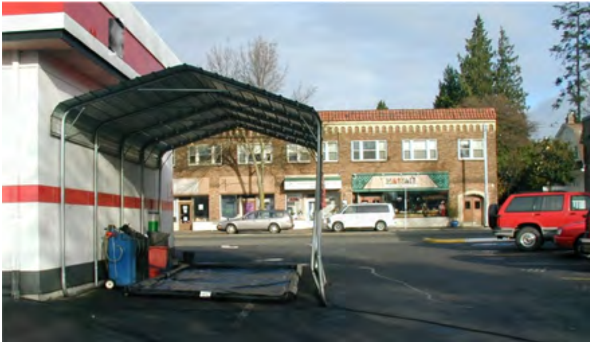
Figure 4.2. - Uncovered Washing Area for Tools, Engines, Equipment, and Portable Objects, with Drains to a Sanitary Sewer, Process Treatment, or a DeadEnd Sump.
