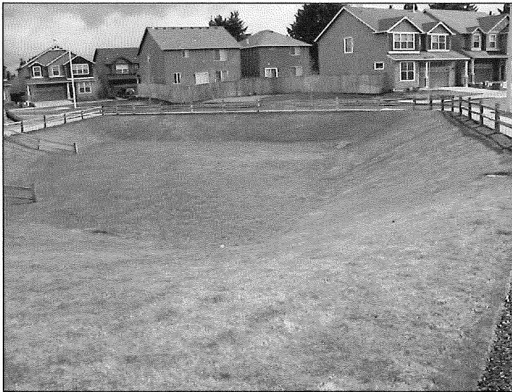
Example of a Manicured Detention Pond
