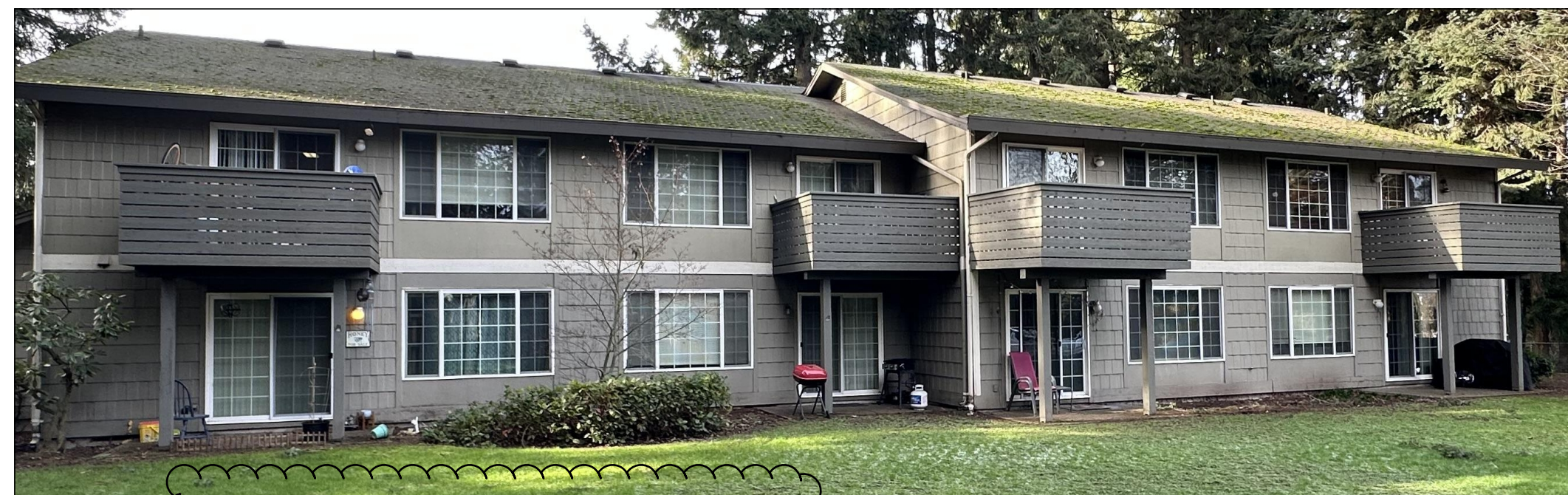
Photos of Existing Conditions
