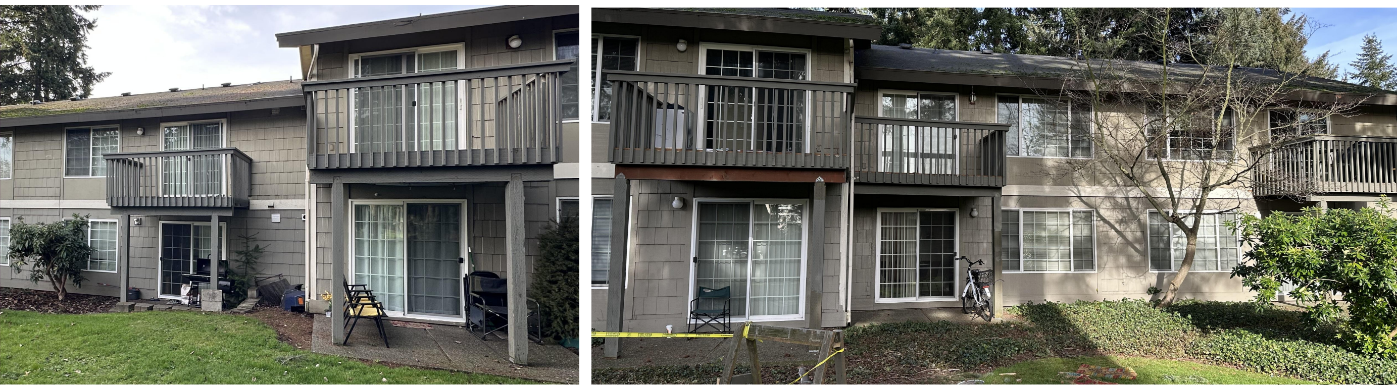
Photos of Existing Conditions
