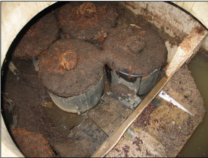
Media Cartridge Filter Vault with Accumulated Sediment
