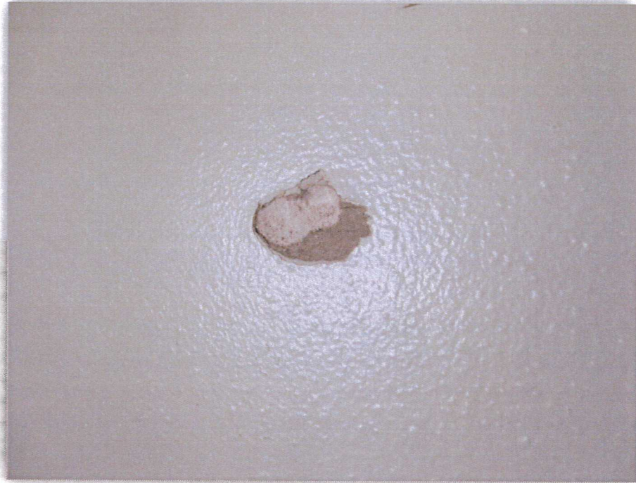
Photo 19: Orange Peel Wall Texture
