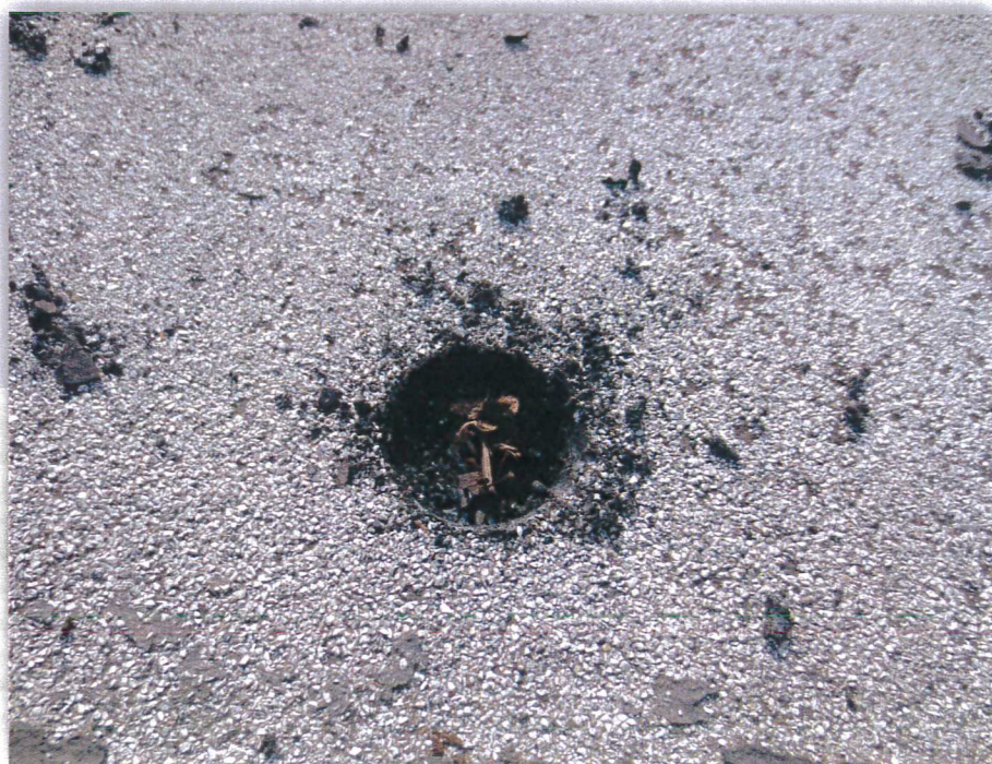
Photo 26: Built Up Roofing
