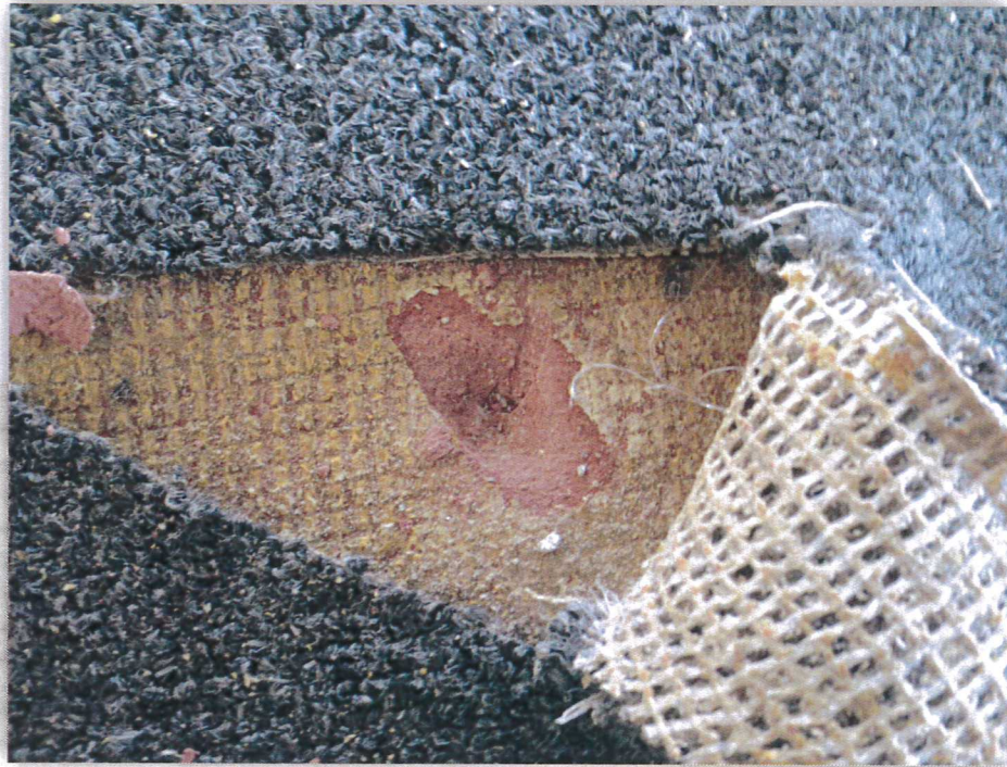
Photo 7: Red Flooring Underlayment
