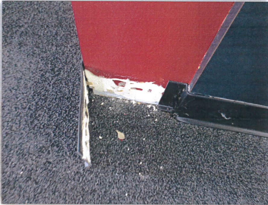
Photo 11: Cove Base Mastic
