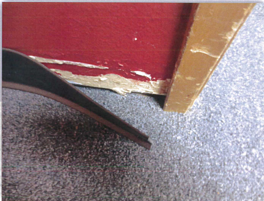
Photo 12: Cove Base Mastic
