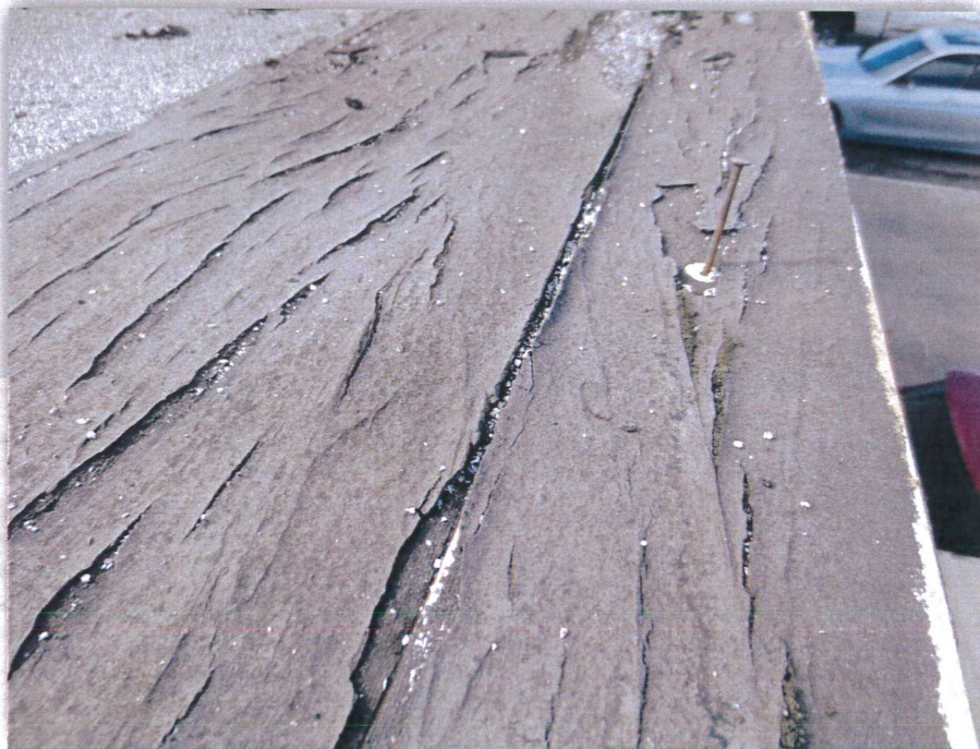
Photo 30: Dark Grey Roofing Mastic
