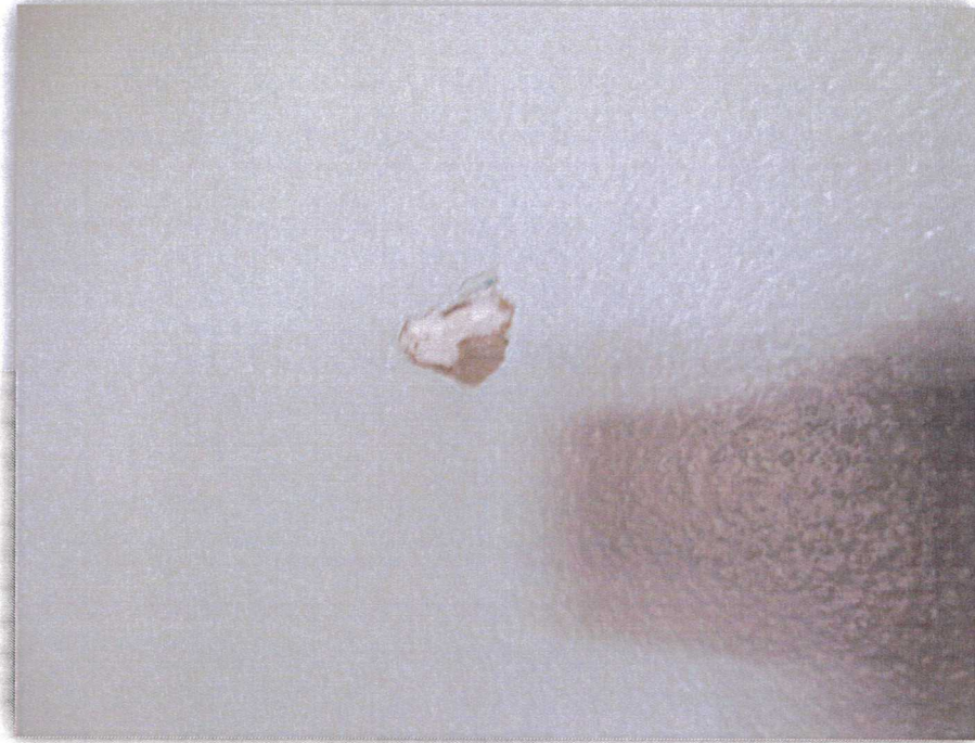
Photo 17: Orange Peel Wall Texture
