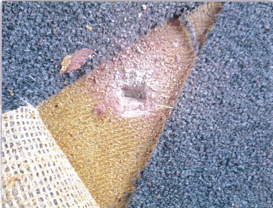
Photo 10: Red Flooring Underlayment
