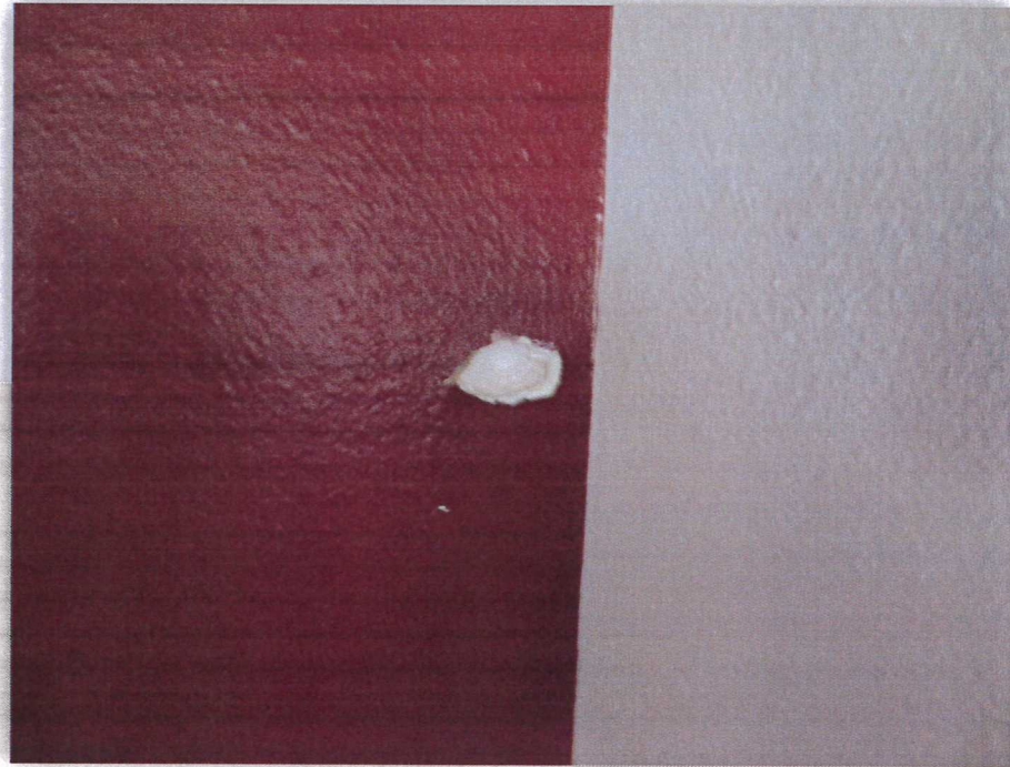
Photo 13: Joint Compound and Drywall
