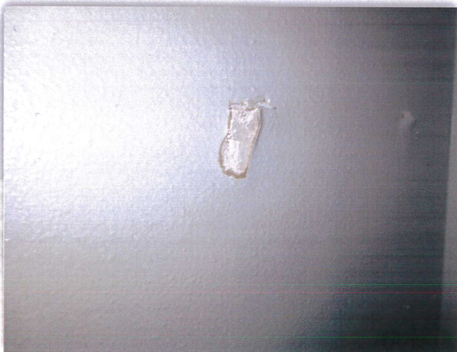
Photo 16: Orange Peel Wall Texture
