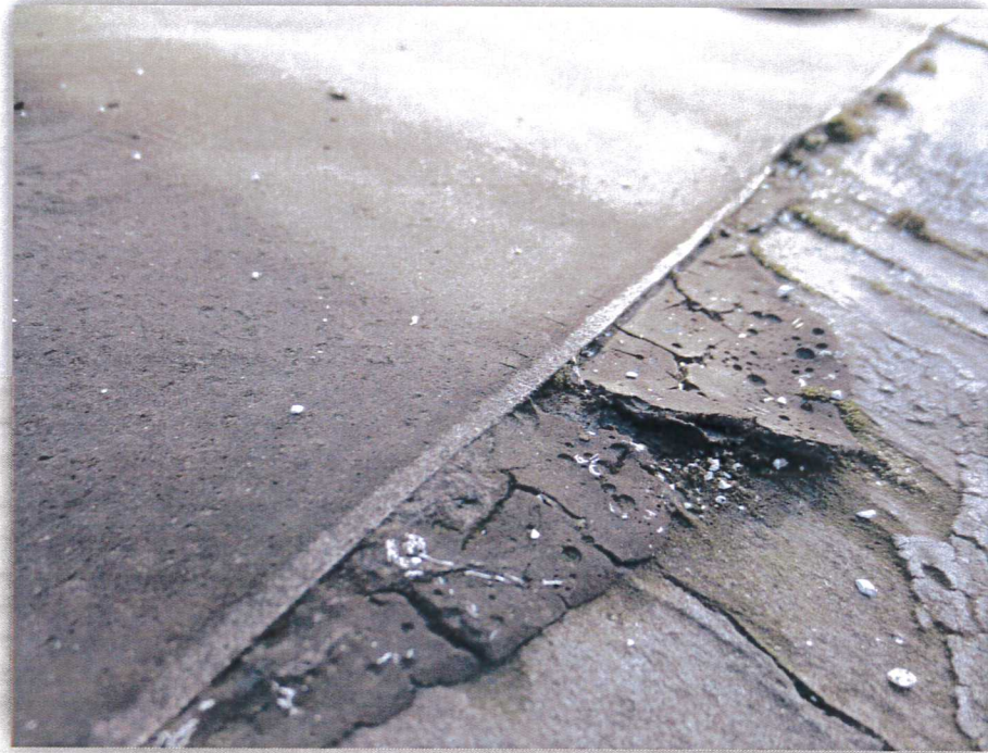
Photo 31: Black Roofing Mastic
