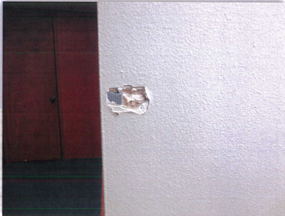
Photo 14: Joint Compound and Drywall
