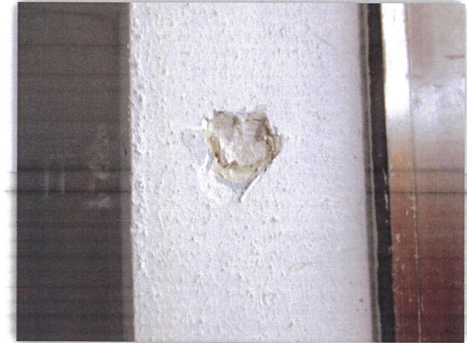
Photo 37: Joint Compound and Drywall
