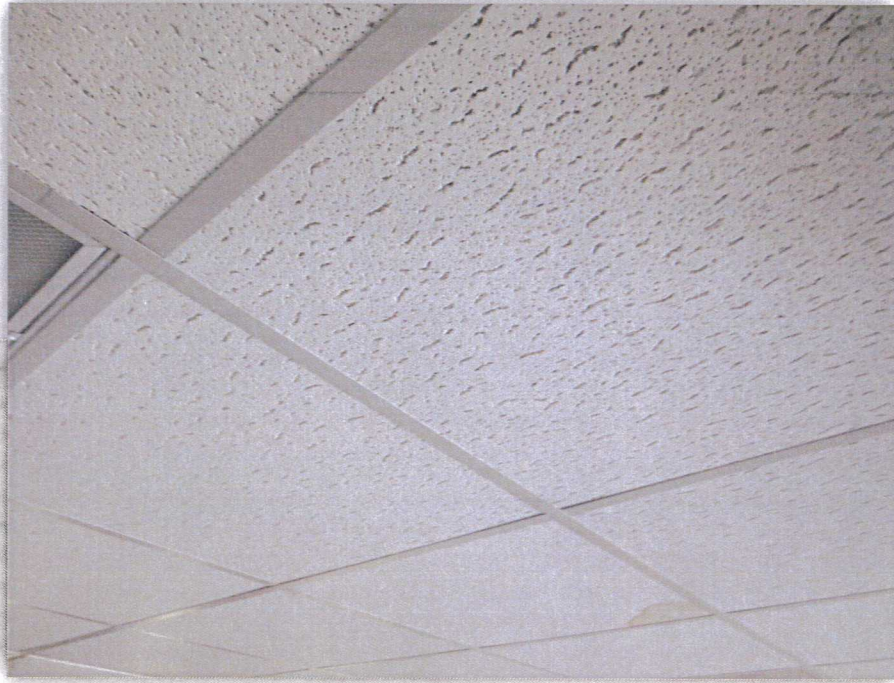
Photo 21: White Suspended Ceiling Tile
