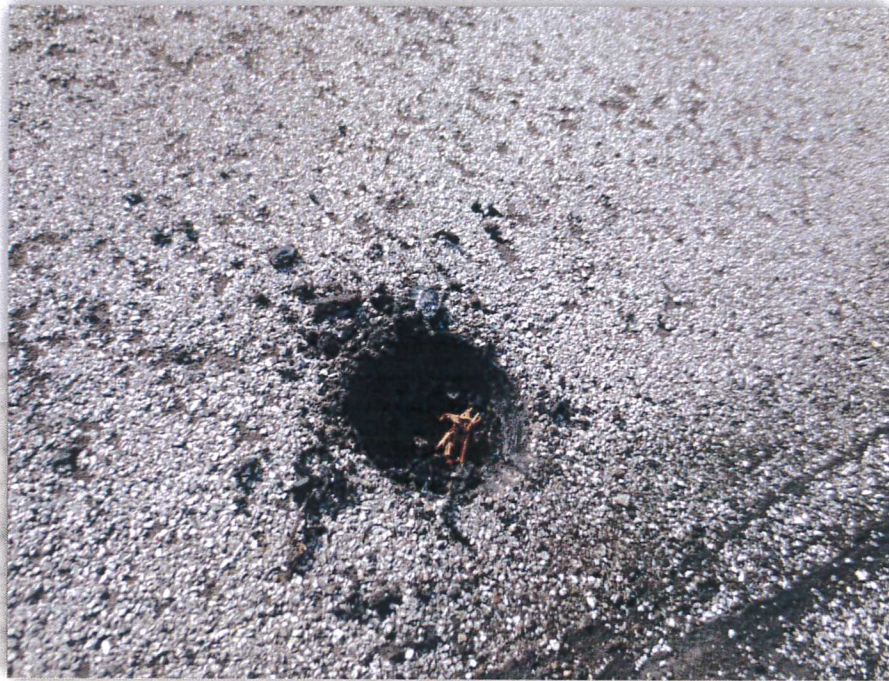
Photo 27: Built Up Roofing
