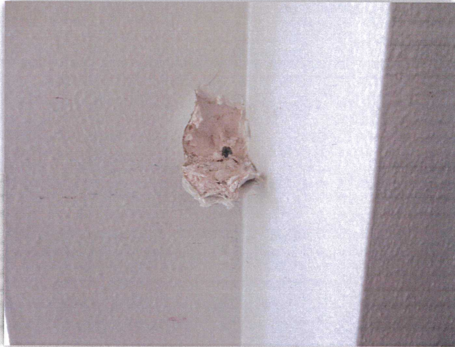
Photo 15: Joint Compound and Drywall
