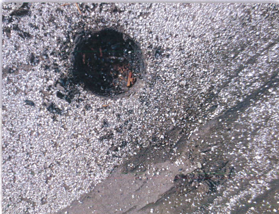
Photo 28: Built Up Roofing
