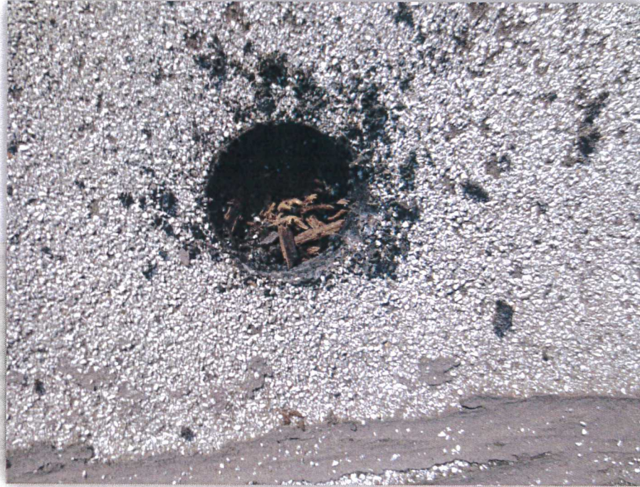
Photo 29: Built Up Roofing
