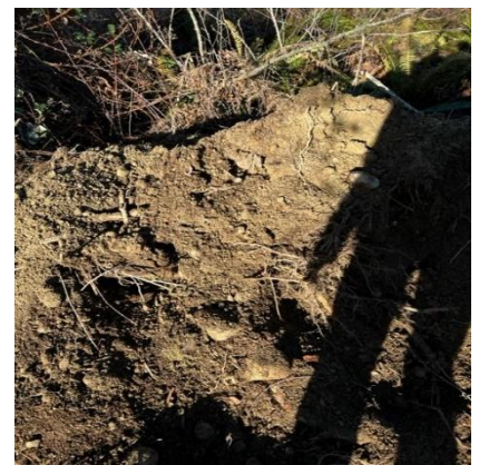
Backfill Test Hole
