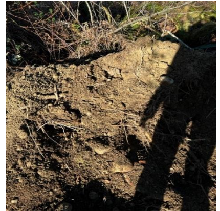
Backfill Test Hole
