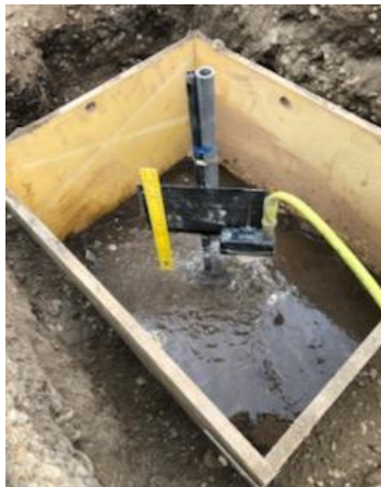
Test Pit Pre-soak at 12-inches
