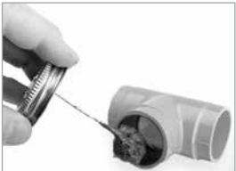
Apply Solvent Cement to Fitting
