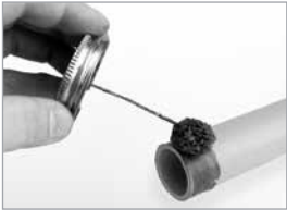
Apply Solvent Cement to Pipe End
