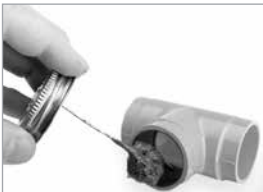
Apply Solvent Cement to Fitting
