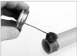
Apply Solvent Cement to Pipe End
