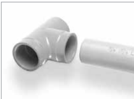
Clean & Fit Pipe & Fitting
