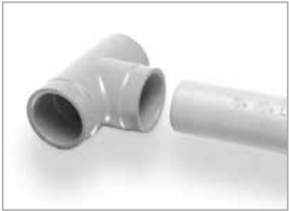
Clean & Fit Pipe & Fitting
