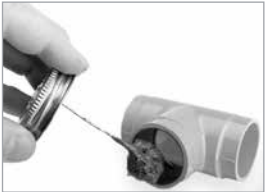
Apply Solvent Cement to Fitting
