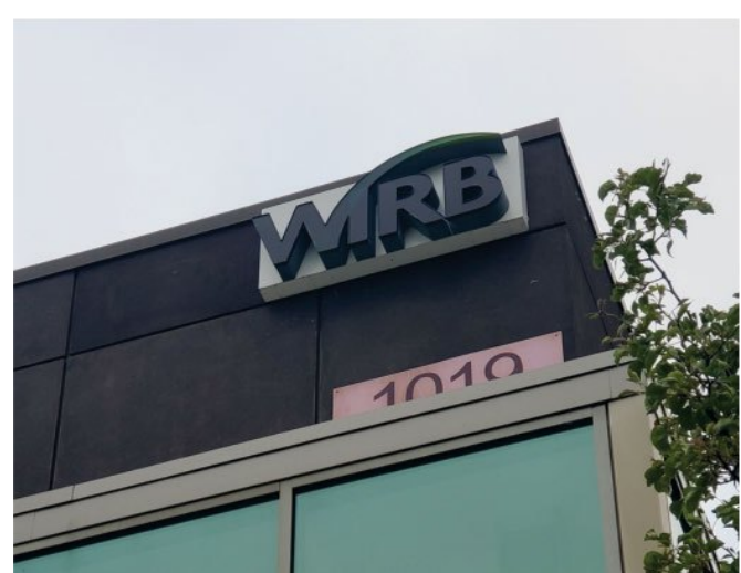
Existing sign to be removed
