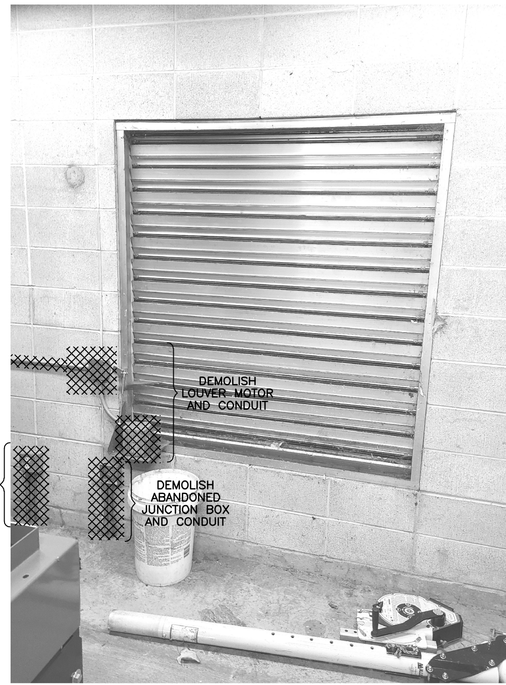
DETAIL 3/E-9 EAST WALL SCALE: NONE
