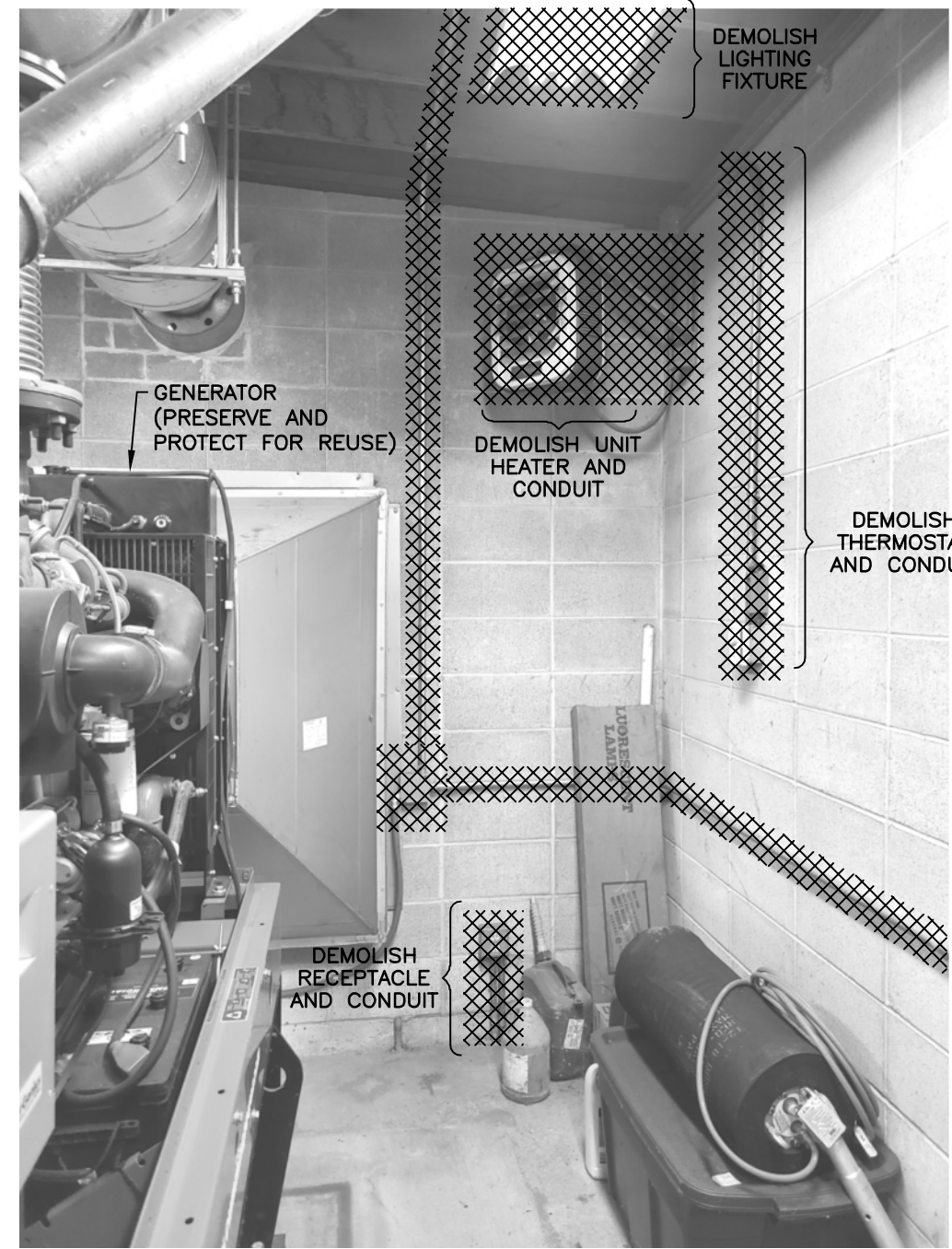
DETAIL 2/E-9 NORTHEAST CORNER SCALE: NONE
