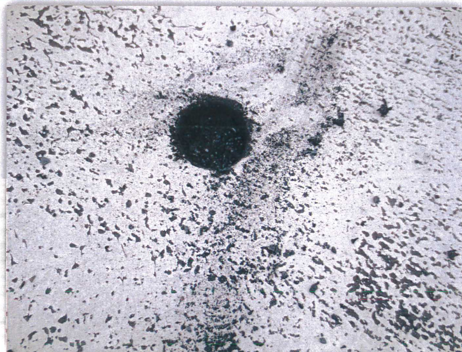
Photo 46: Built Up Roofing
