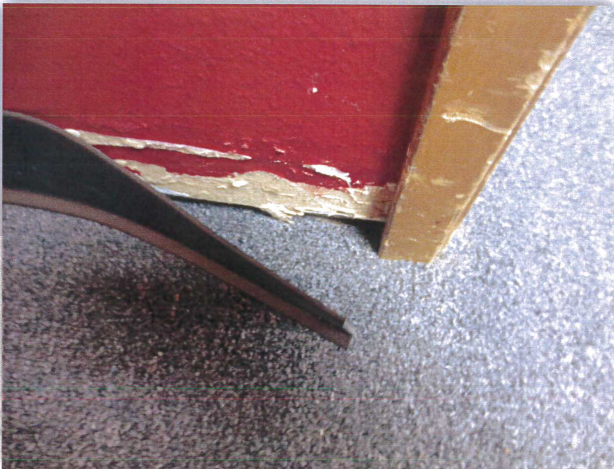
Photo 12: Cove Base Mastic
