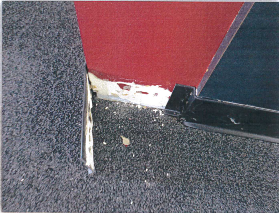
Photo 11: Cove Base Mastic
