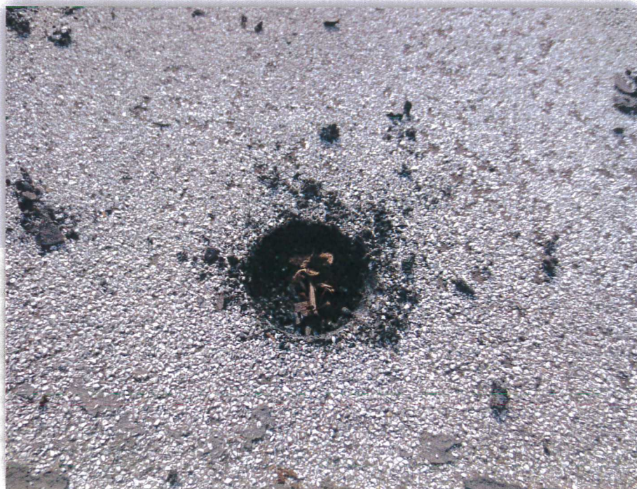
Photo 26: Built Up Roofing
