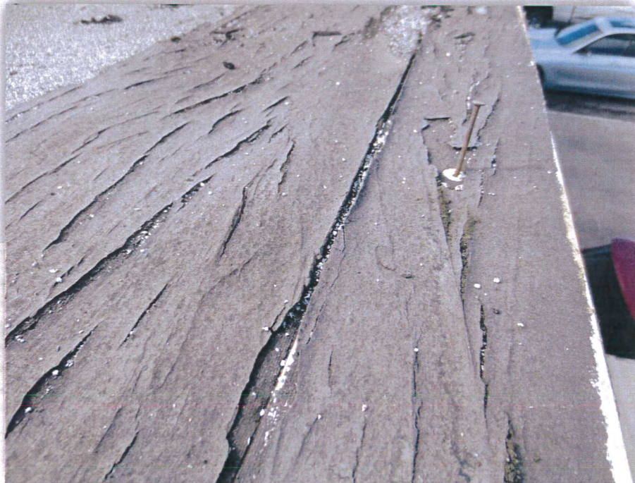
Photo 30: Dark Grey Roofing Mastic
