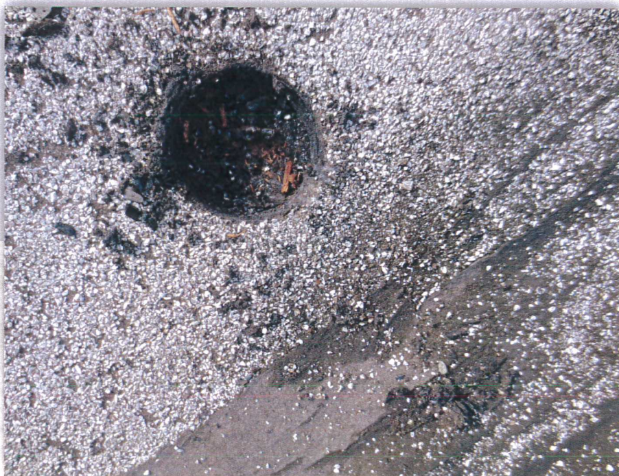
Photo 28: Built Up Roofing
