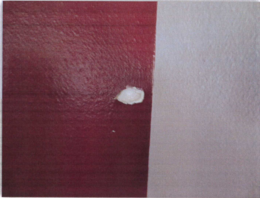
Photo 13: Joint Compound and Drywall
