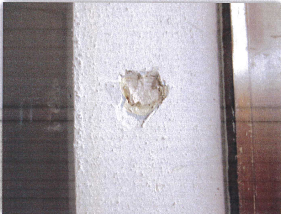
Photo 37: Joint Compound and Drywall
