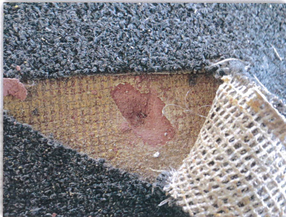
Photo 7: Red Flooring Underlayment
