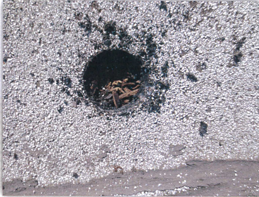
Photo 29: Built Up Roofing
