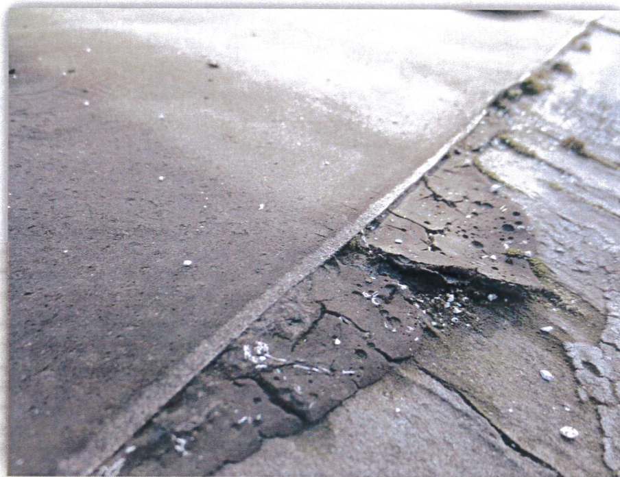
Photo 31: Black Roofing Mastic
