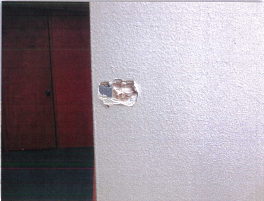
Photo 14: Joint Compound and Drywall
