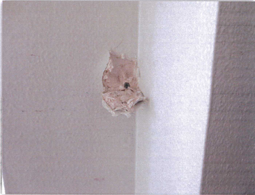
Photo 15: Joint Compound and Drywall
