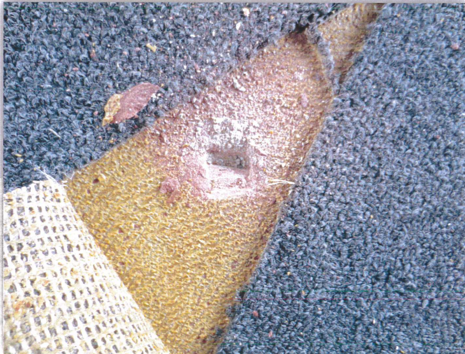
Photo 10: Red Flooring Underlayment
