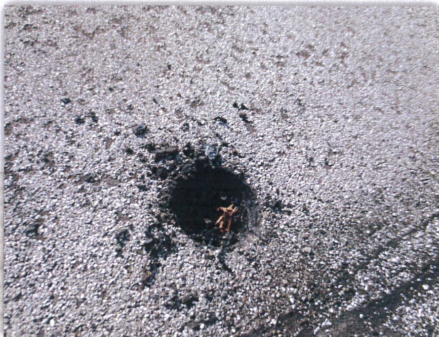
Photo 27: Built Up Roofing
