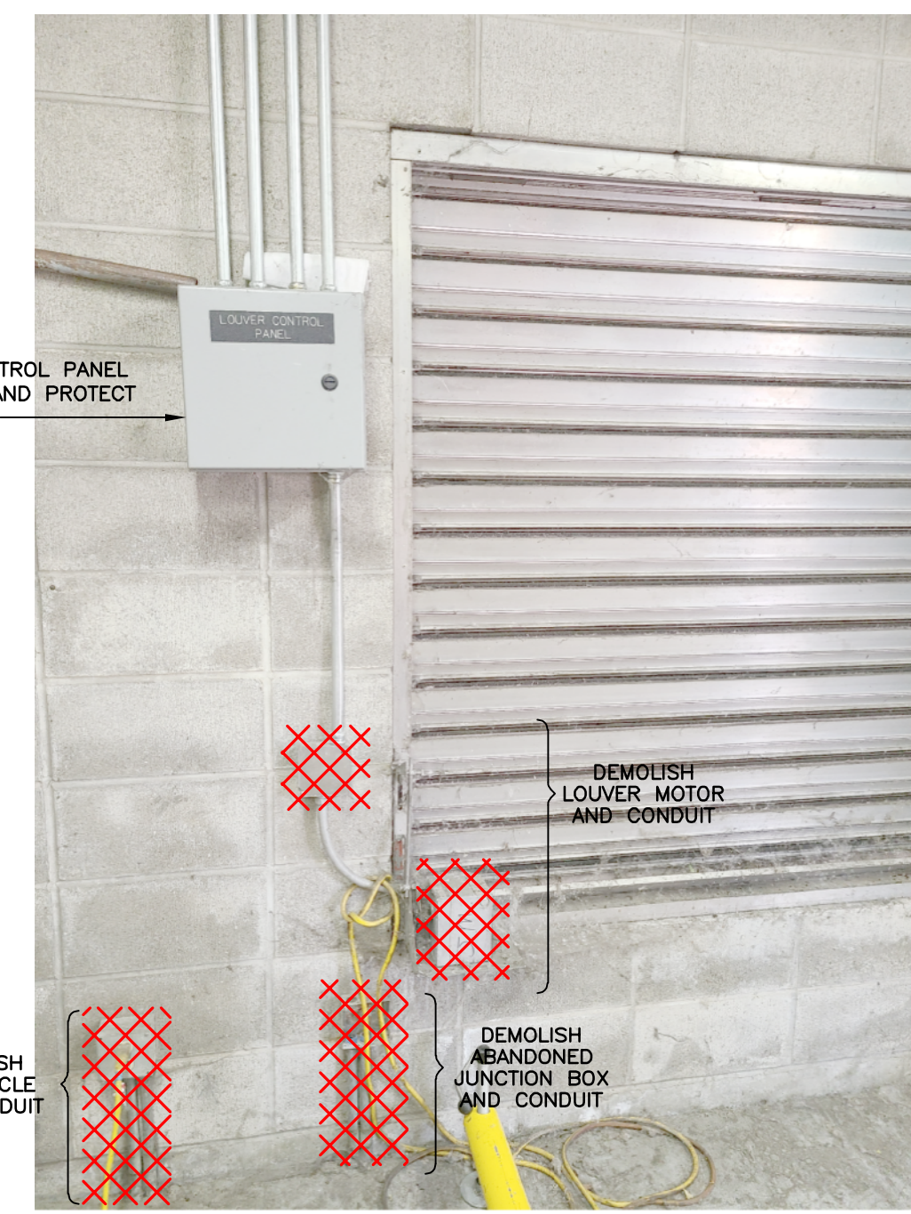
DETAIL 4/E-9 SOUTH WALL SCALE: NONE
