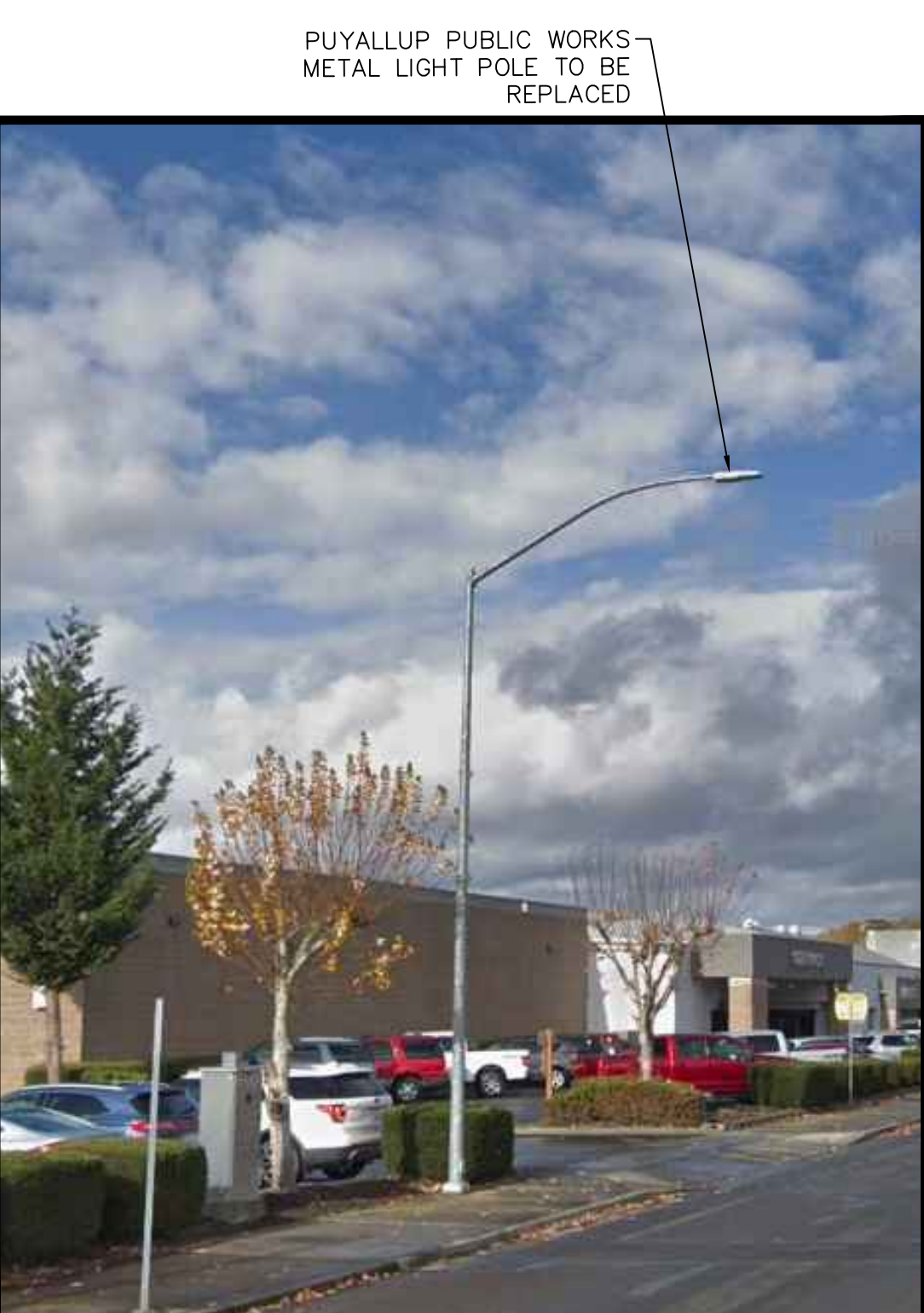
EXISTING POLE ELEVATION - LOOKING NORTHWEST
