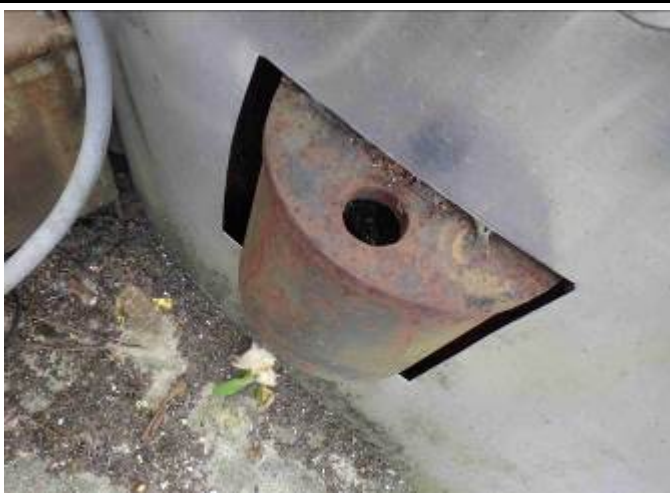
Missing Anchor Bolt
