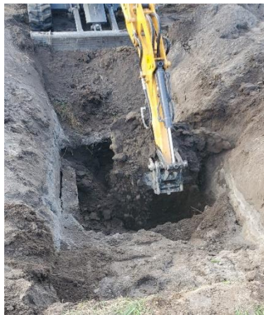
Over Excavate to Verify if Groundwater is Mounding
