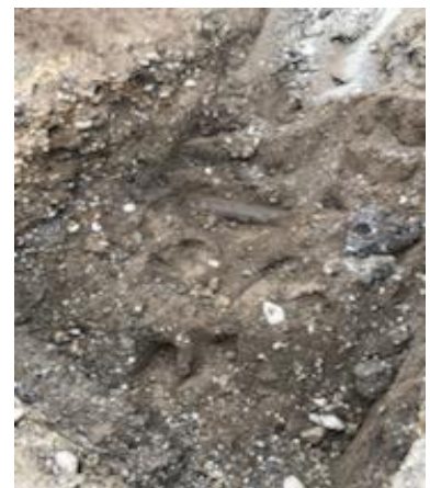
Backfill Test Hole & Install Groundwater Monitoring Pipe
