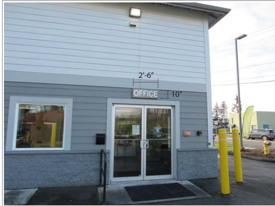
Note: PSG to remove the existing OFFICE wall sign, cap electrical and remediate the wall.
