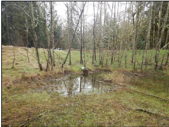
Figure 2. Stormwater Pond Conveyance Features
