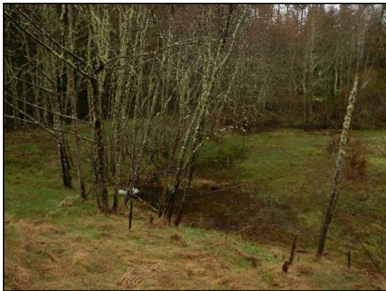
Figure 3. Stormwater Pond Conditions
