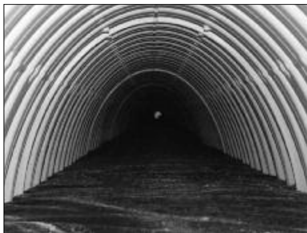
Looking down the Isolator Row.
