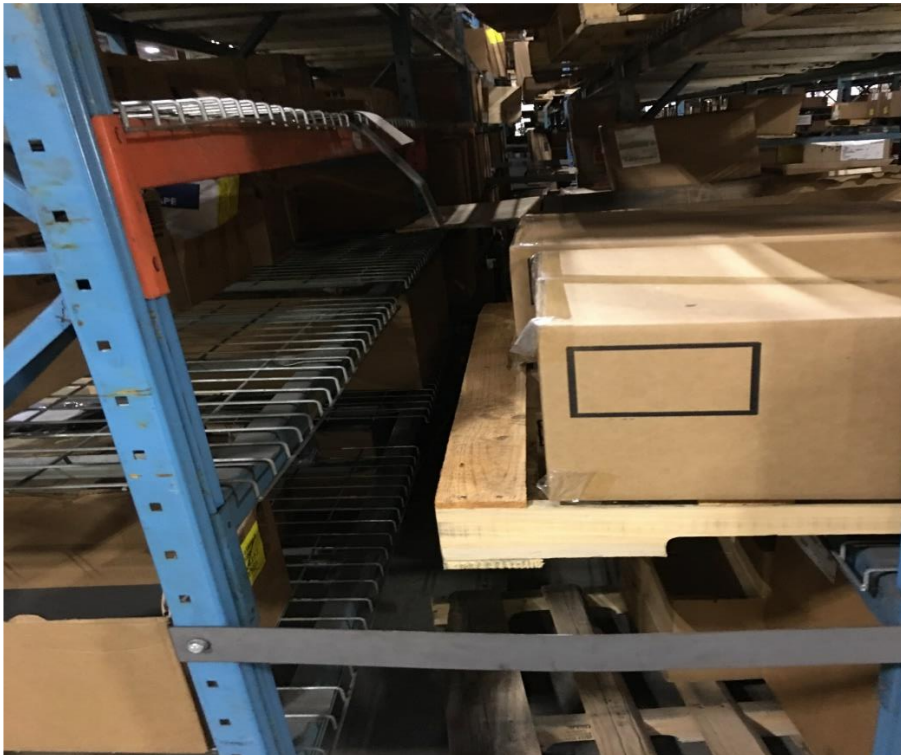
Picture 2 – Flue in Rack
