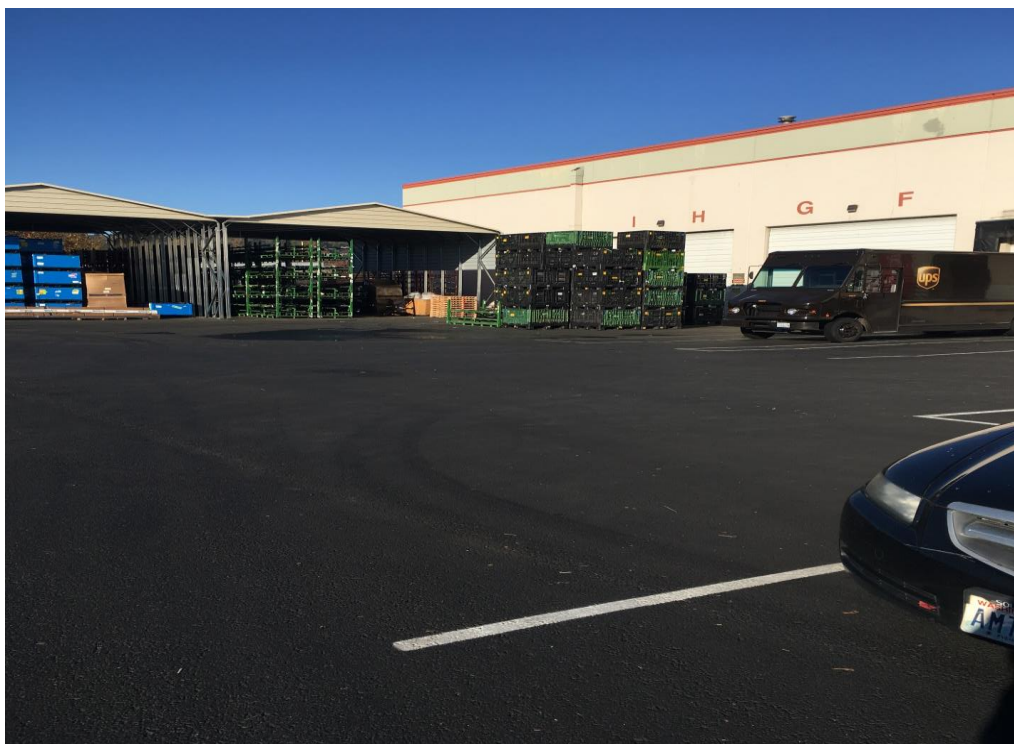
Picture 2 – Exterior Combustibles
