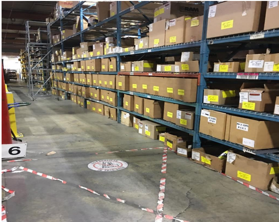
Picture 3 – No Flues with Box Loads
