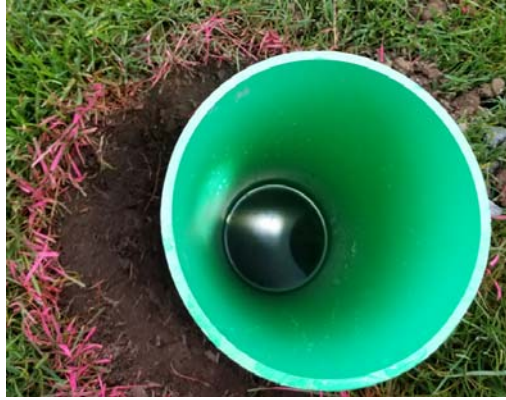
Photo 3: Test Pit 2 during percolation period.
