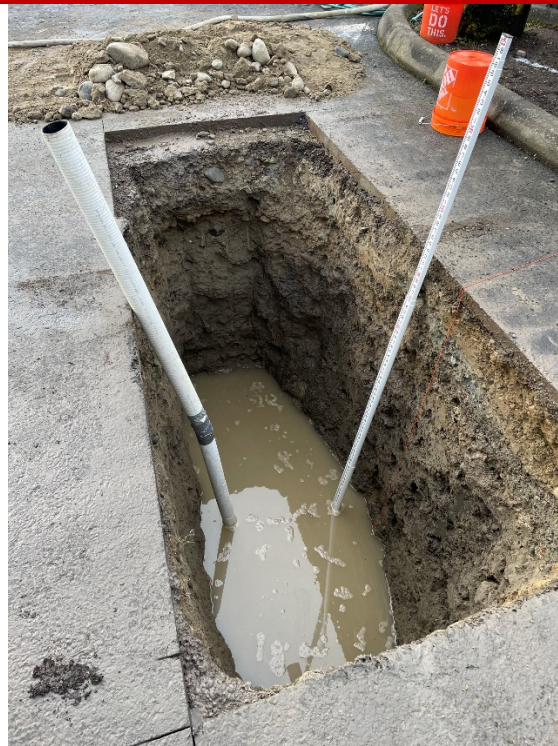
Photo 3: Infiltration Testing at PIT-01
