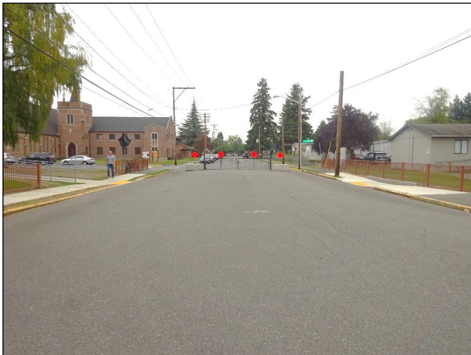
WESTERLY VIEW OF SUBJECT PROPERTY (WEST MAIN)
