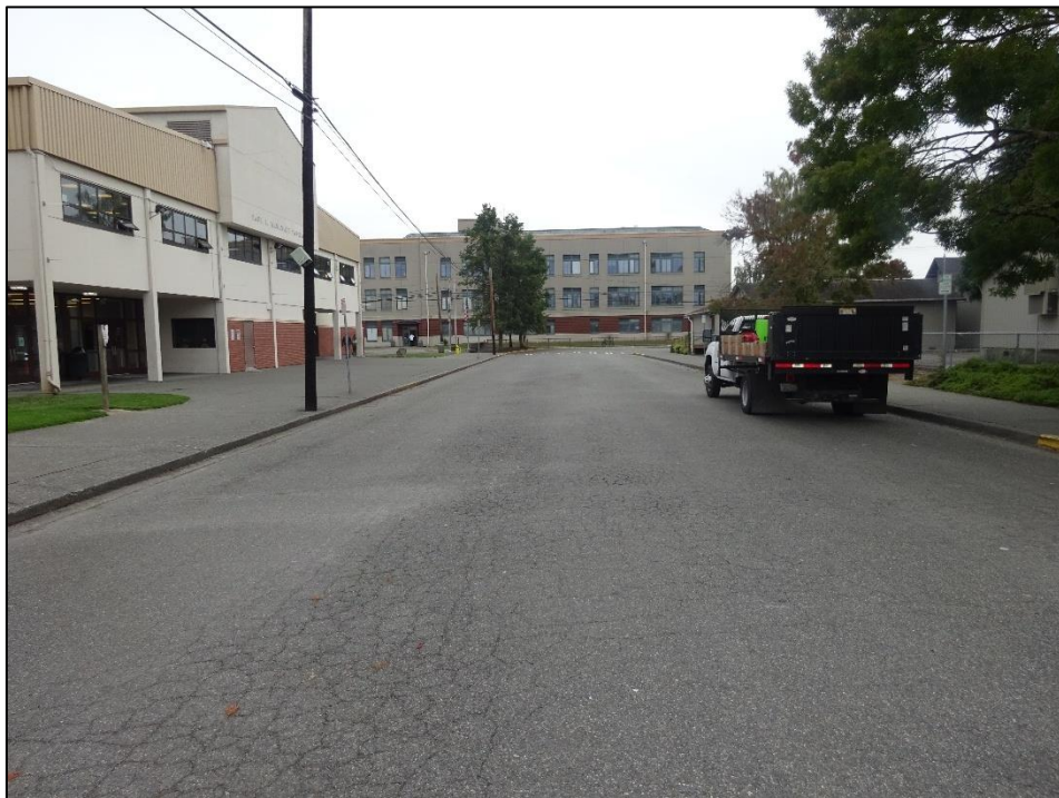
SOUTHERLY VIEW OF SUBJECT PROPERTY (7 TH STREET NW)
