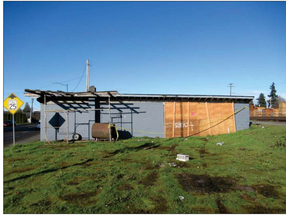
EAST ELEVATION OF SUBJECT BUILDING
