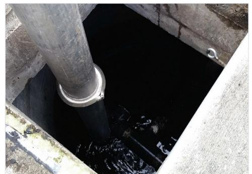
Jet Vactoring Through Access Hatch
