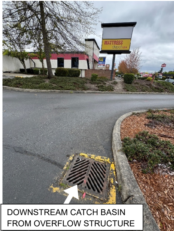
Photograph 1 – Existing Downstream Catch Basin Within South Access To Be Replaced – Discharge From Overflow Structure
