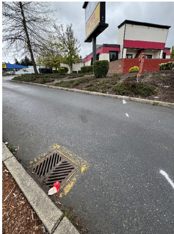
Photograph 2 – Existing Downstream Catch Basin Within South Access – Upstream of S Meridian Tie-In
