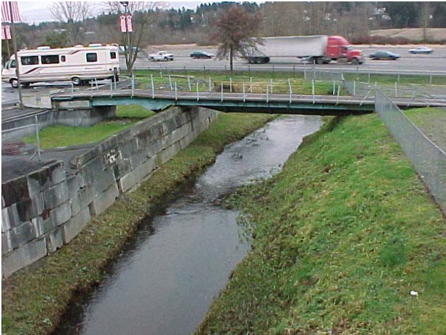
Existing Hylebos Creek in the Vicinity of I-5
