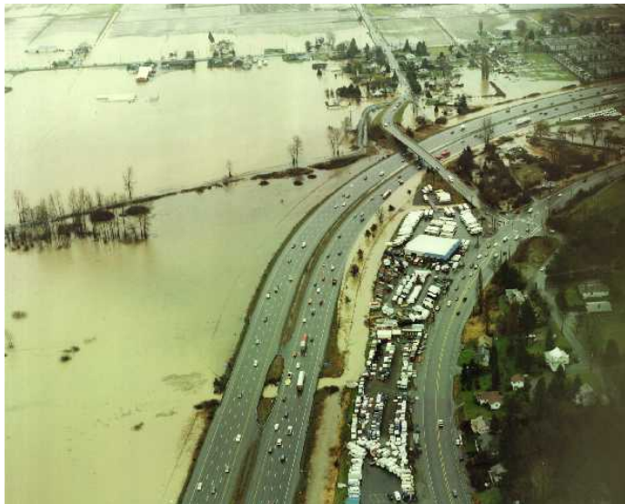
Flooding in February 1996 at Hylebos Creek and I-5
