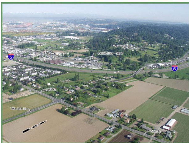
Current view of I-5 at the Fife Curve
