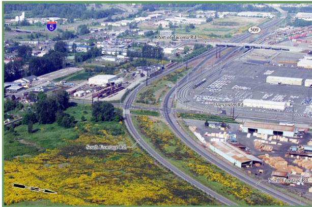
Current view along SR 509
