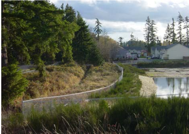
Conventional stormwater ponds sometimes encroach into riparian buffers of the streams they are intended to protect.
