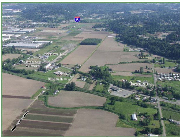
Current view of Valley Avenue East
