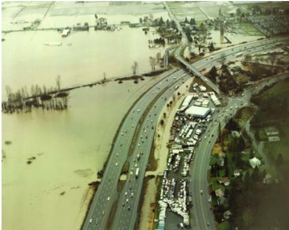
Flooding along I-5 at Hylebos Creek in February 1996.
