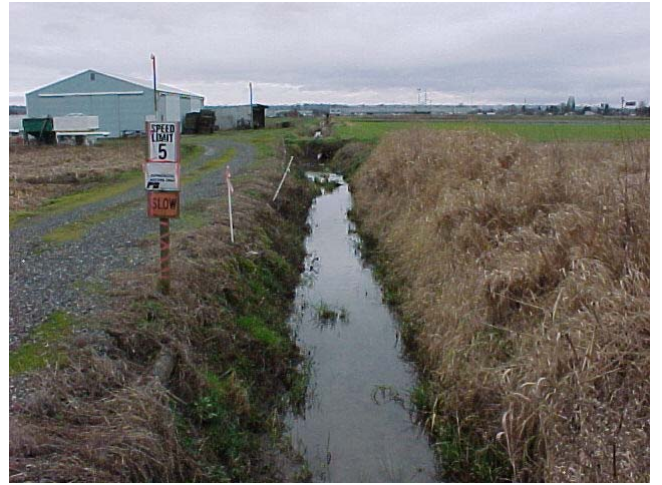
Existing Surprise Lake Drain West of Freeman Road
