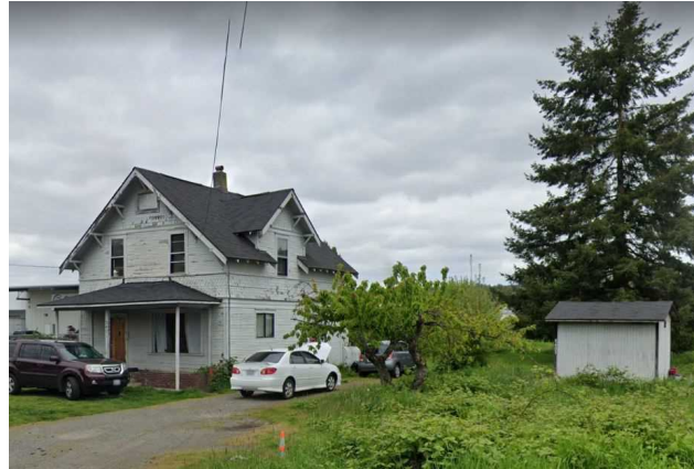
2401 Inter Ave facade, east elevation, and out bldg
