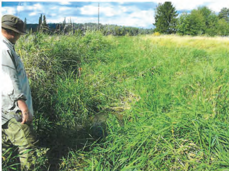
Photo #6: Looking north at slowly flowing water in the small drainage ditch as shown in Photo #8 is due to clogging by dense vegetation (Reed Canary Grass). (Taken 9/28/07)
