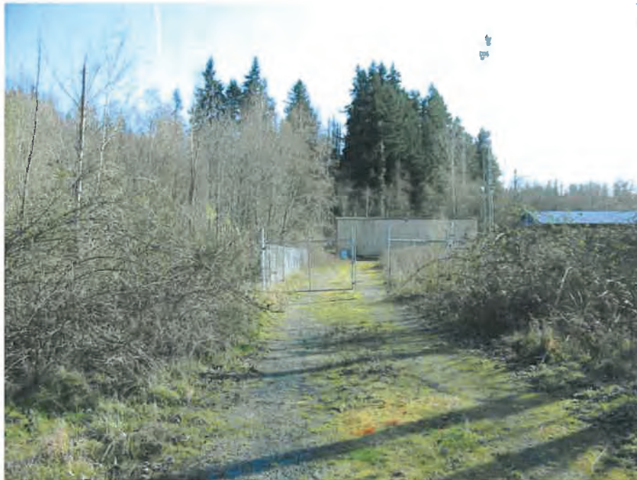
Photo #12: Looking south from within the eastern part of the project site along the gravel road that is constructed in the surveyed location shown on Figure 7. Note the storm water detention pond is on the left in the photo, and the fenced area in the background is within the project site. (IMG-032, 3/4/20)
