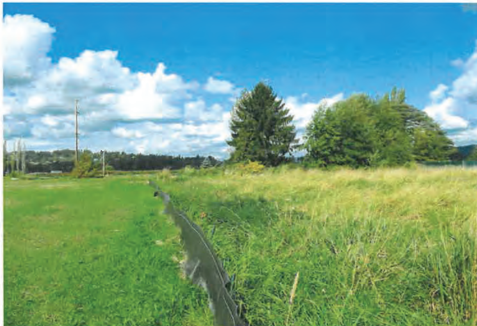
Photo #2: Looking north along the ditch-line pictured in photo #1. The ditch flows along (just outside) the east property line. The silt fence runs along the property line to protect the ditch from onsite surface runoff in accordance with the City of Puyallup requirements for the approved site development permit.
