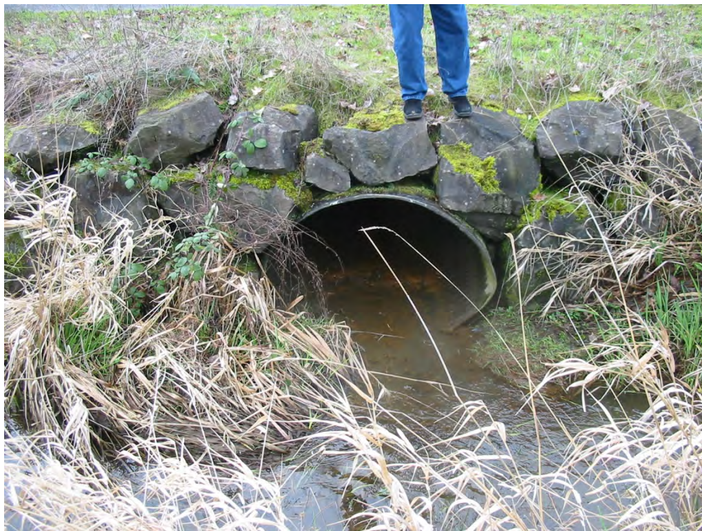
Photo #14: Looking at the outlet (downstream end) of the CMP Arch culvert under Pioneer Way where Wetland “A” drains unconstricted into “Deer Creek”. Note that the creek was in the foreground flowing from left to right in this photo. (Taken 2/15/13)
